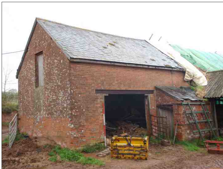
Plate 14: The mid-late 19th-century stable, looking east (2m scale)
