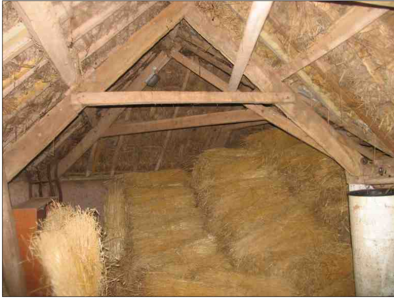
Plate 7: The roof over the dairy, looking south
