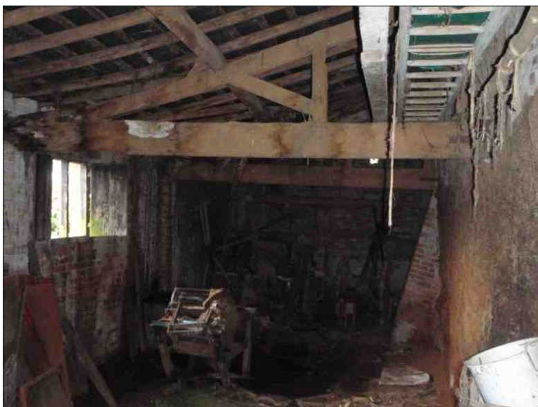
Plate 9: Internal view of the root house, looking south
