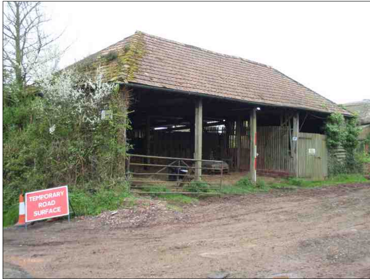
Plate 16: The wagon shed, looking southwest
