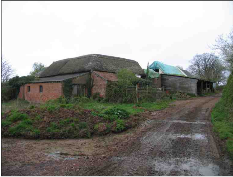
Plate 1: The dairy with attached root store (centre and left) and threshing barn with attached lean-to beyond to the right, looking southwest (2m scale)
