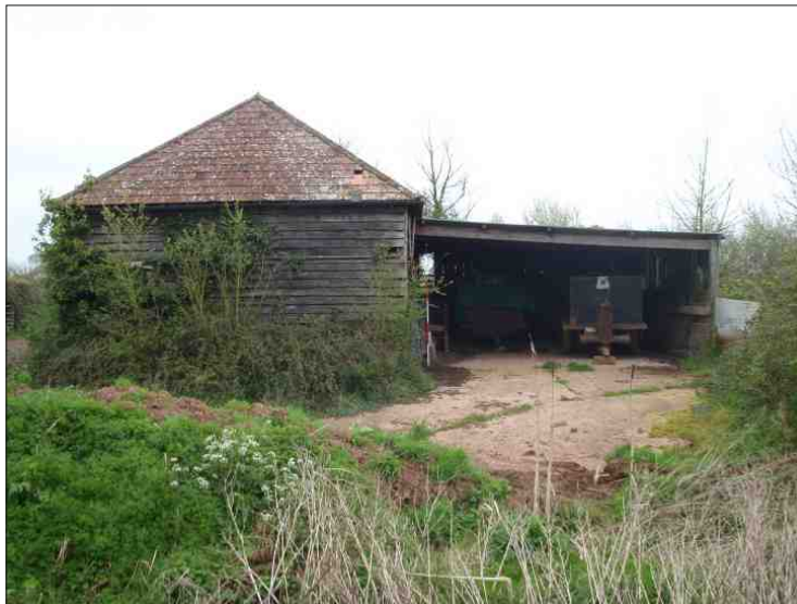
Plate 17: The wagon shed and attached lean-to, looking northeast
