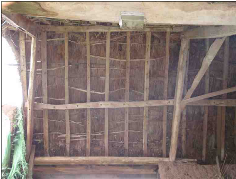
Plate 8: The roof over the dairy, looking north
