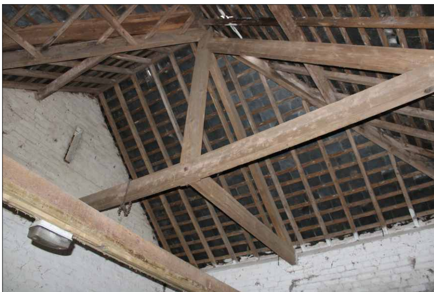
Plate 12: Roof structure of root house, looking west
