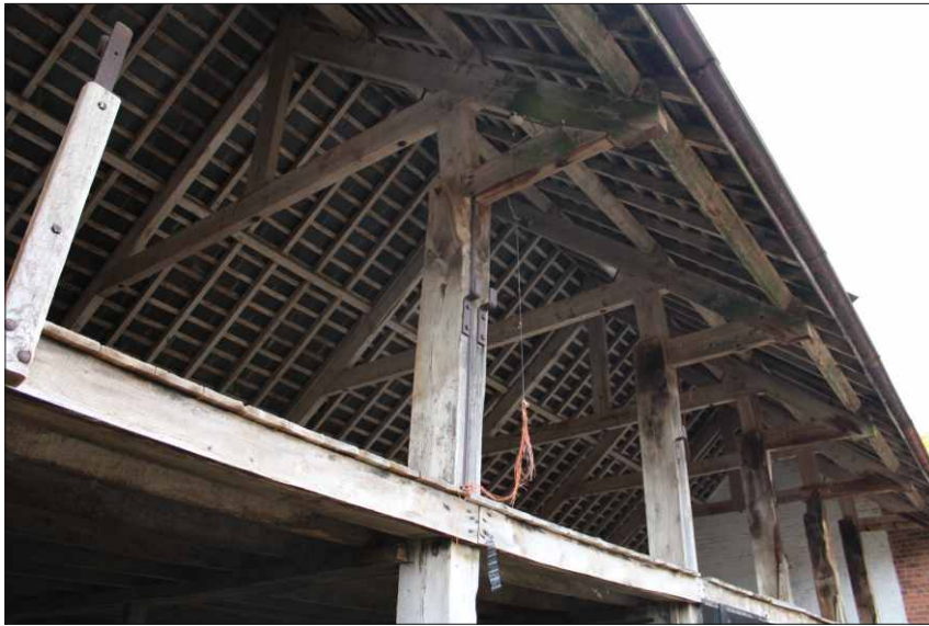
Plate 10: Roof structure of top cattle building, looking northwest
