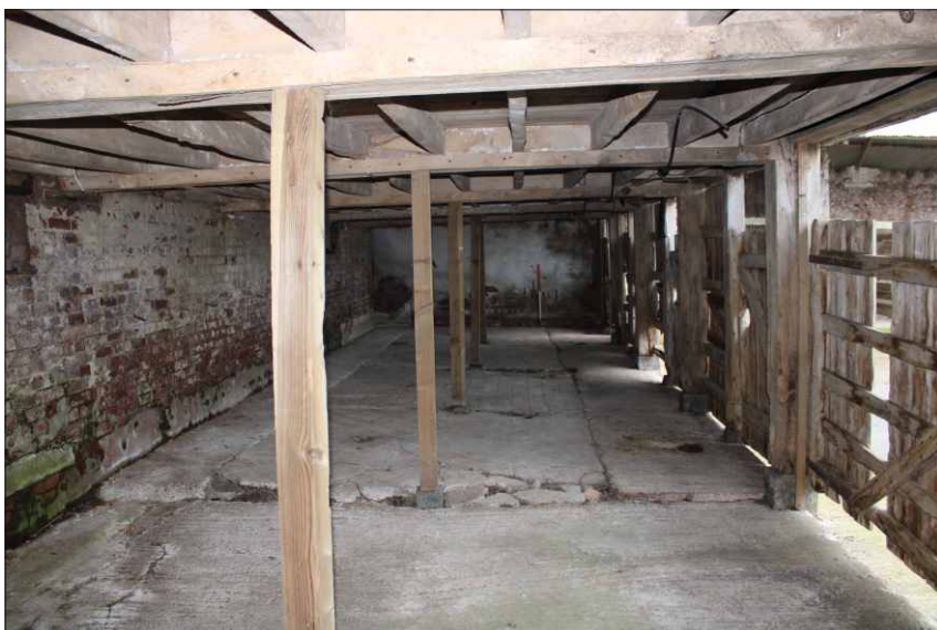
Plate 9: Internal view of top cattle building, looking north (1m scale)
