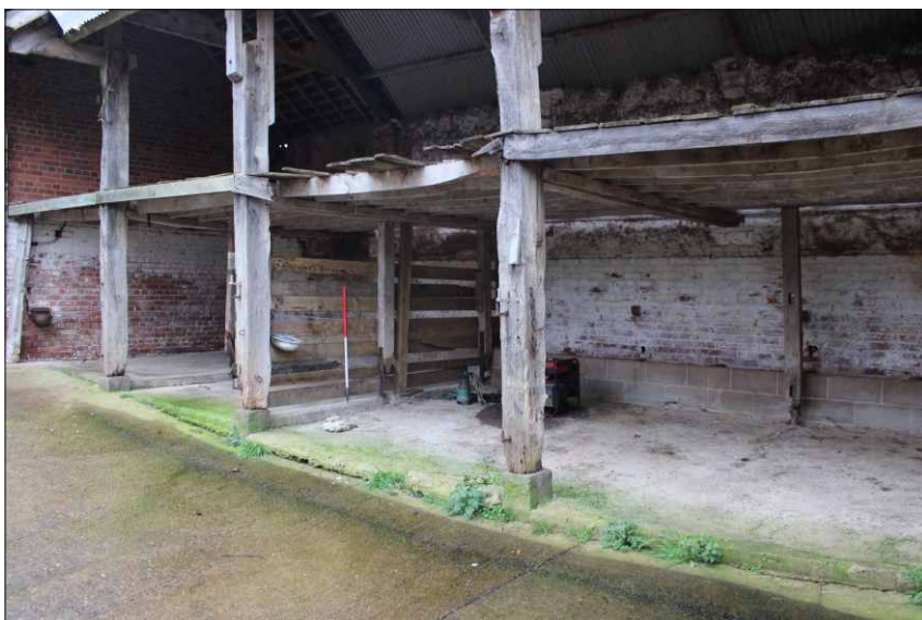
Plate 15: Internal view of far side cattle building, looking northwest (1m scale)
