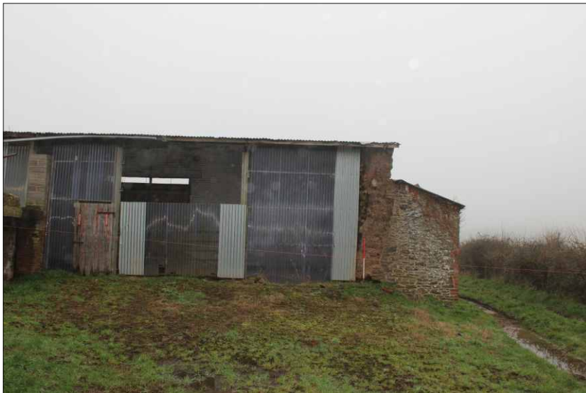
Plate 17: South elevation of the threshing barn, looking north (1m scale)
