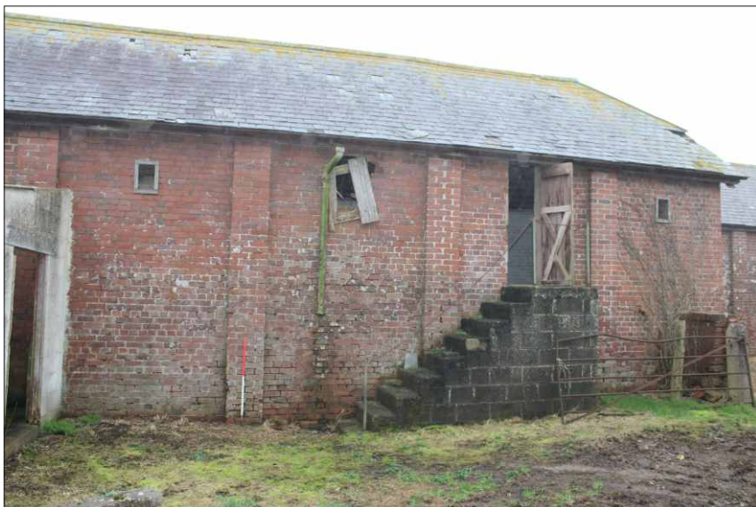
Plate 3: West elevation of the stables, looking east (1m scale)
