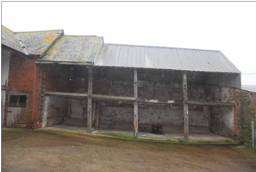
Plate 14: South elevation of far side cattle building, looking north (1m scale)
