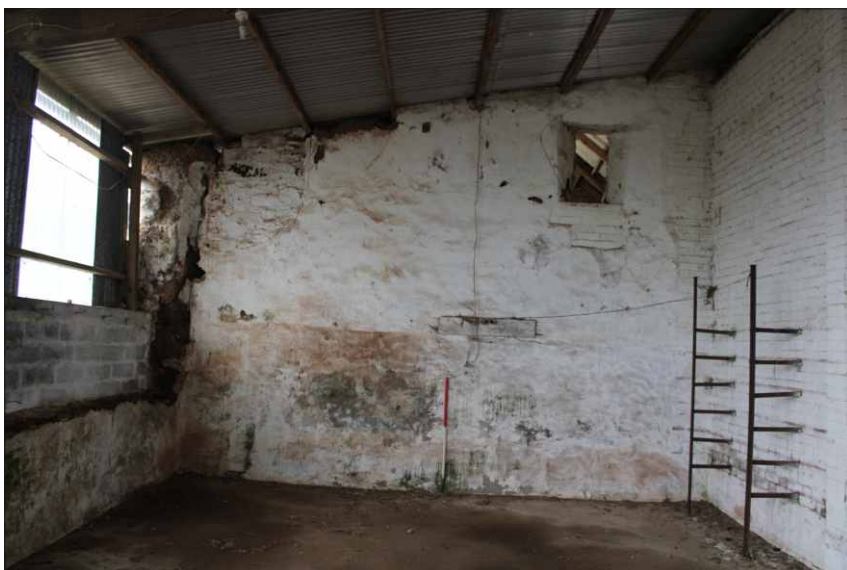
Plate 18: Internal view of threshing barn, looking west (1m scale)
