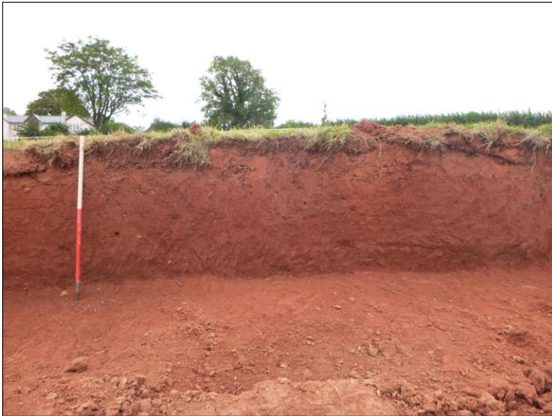
Plate 2: Representative view of excavated easement to northeast of Groper's Lane (scale 1m)
