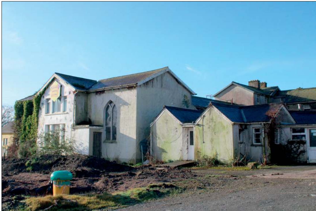
Plate 16: The east elevation of the east range, looking southwest
