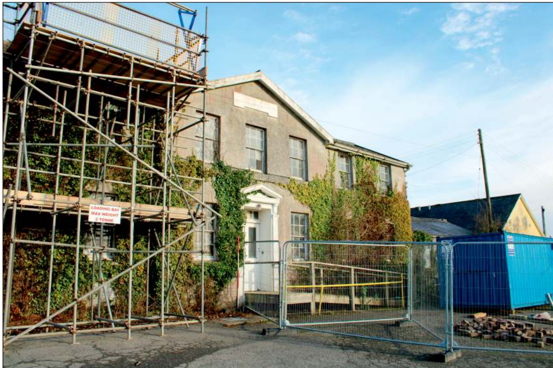
Plate 2: The central section of the south range, looking northeast (2m scale)
