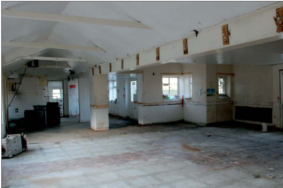
Plate 18: The open-plan north section of the east range, looking north (1m scale)
