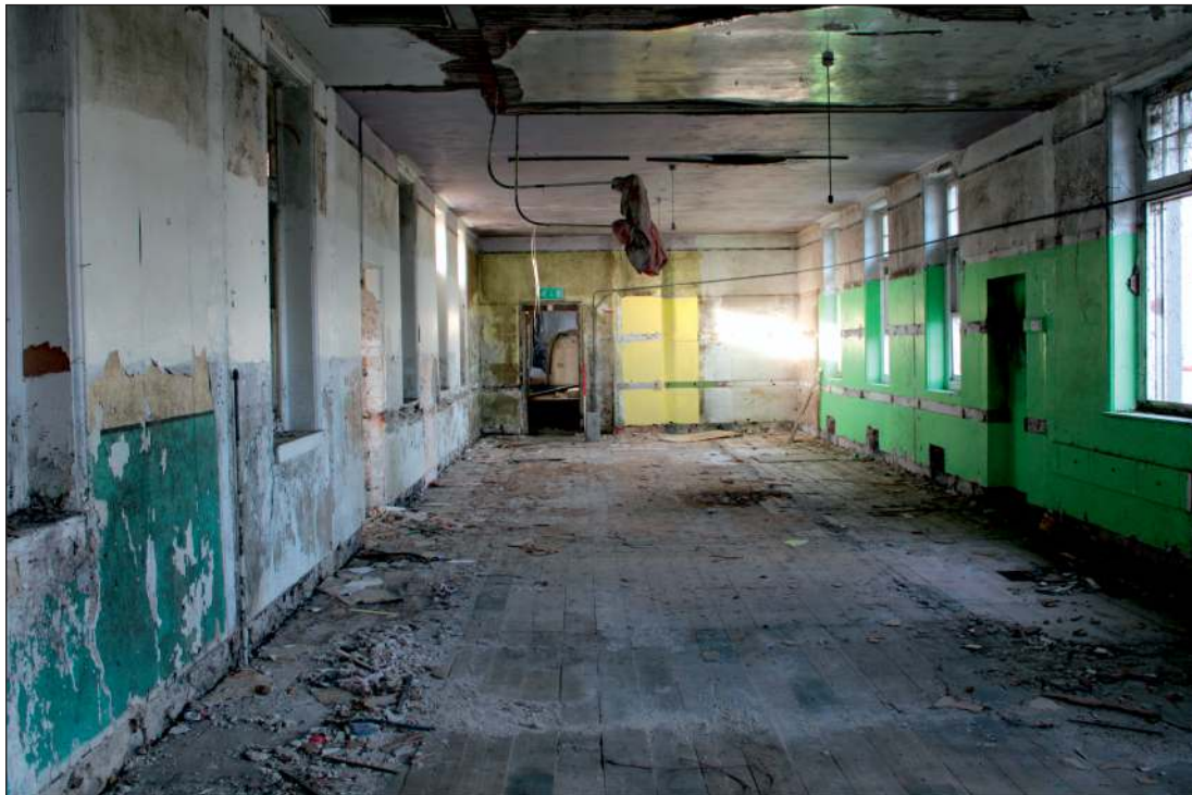
Plate 22: The first floor of the north range, looking north (1m scale)
