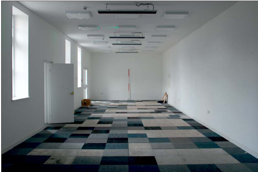
Plate 21: The ground floor of the north range, looking north (2m scale)
