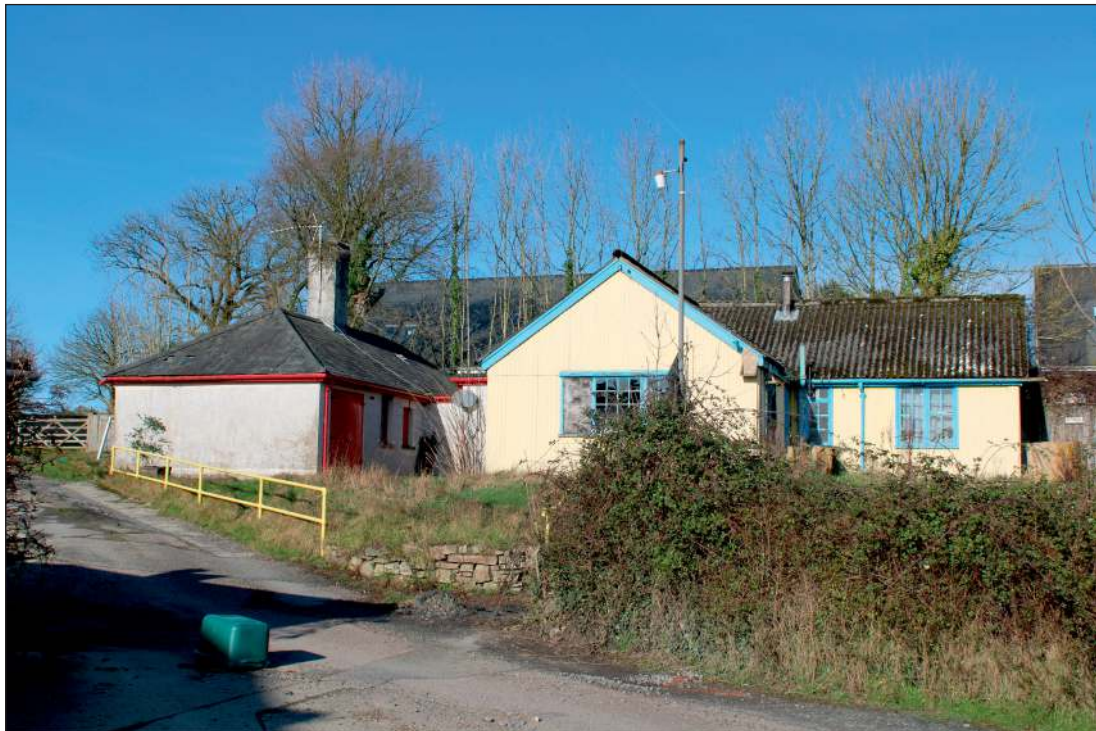
Plate 24: The isolation block, looking north
