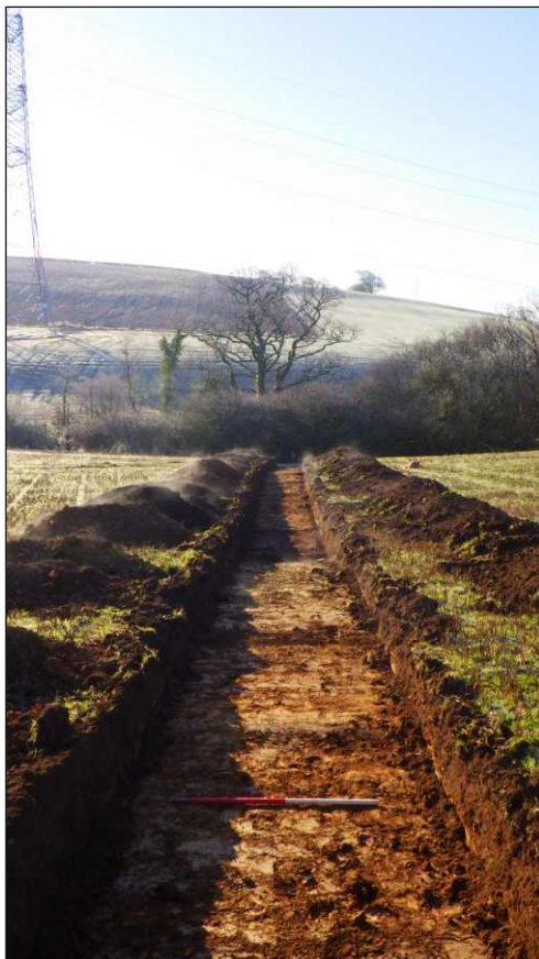
Plate 3: Trench 3 following excavation, looking to south (1m scale)
