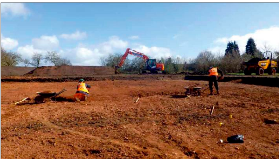
Plate 6: View of excavation area, looking northeast
