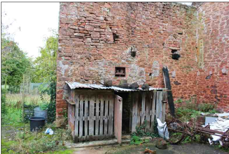
Plate 11: The east end of the threshing barn showing openings, end-bearing box, and evidence for a partial first floor, looking northeast
