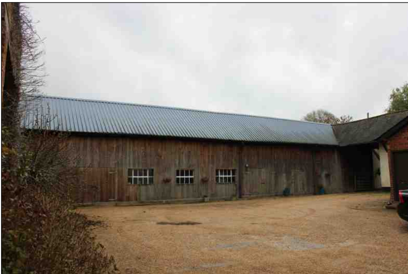
Plate 2: The west elevation of the east range, looking southeast
