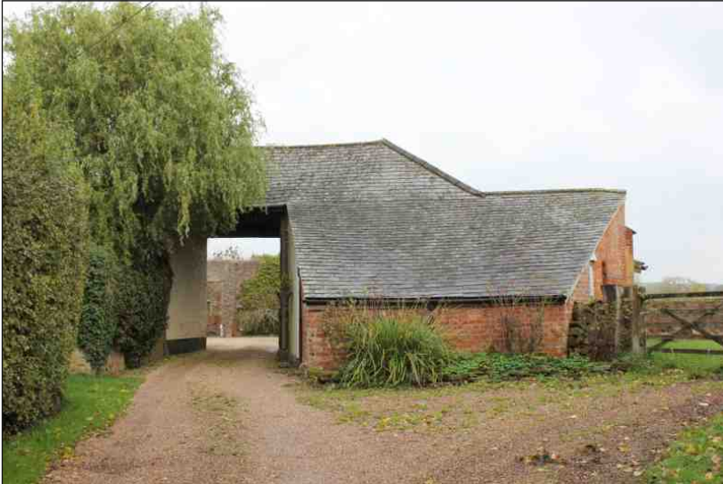
Plate 1: The entrance to the farmyard showing the covered passage and brick extension to the east range, looking north
