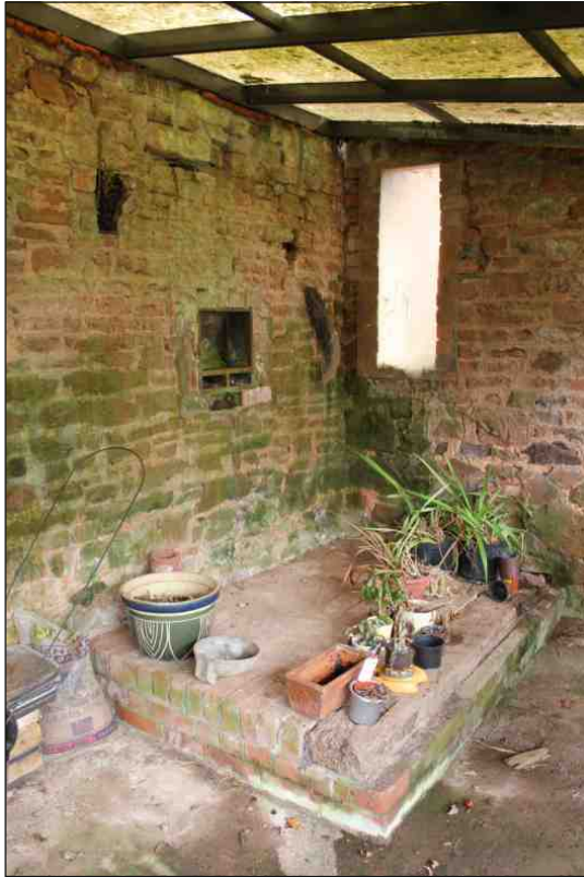
Plate 13: The west barn in the north range showing the end-bearing box, associated opening for a belt, and machine base, looking northeast
