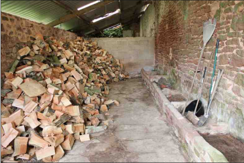
Plate 7: The north end of the attached structure to the east range shippen, looking south
