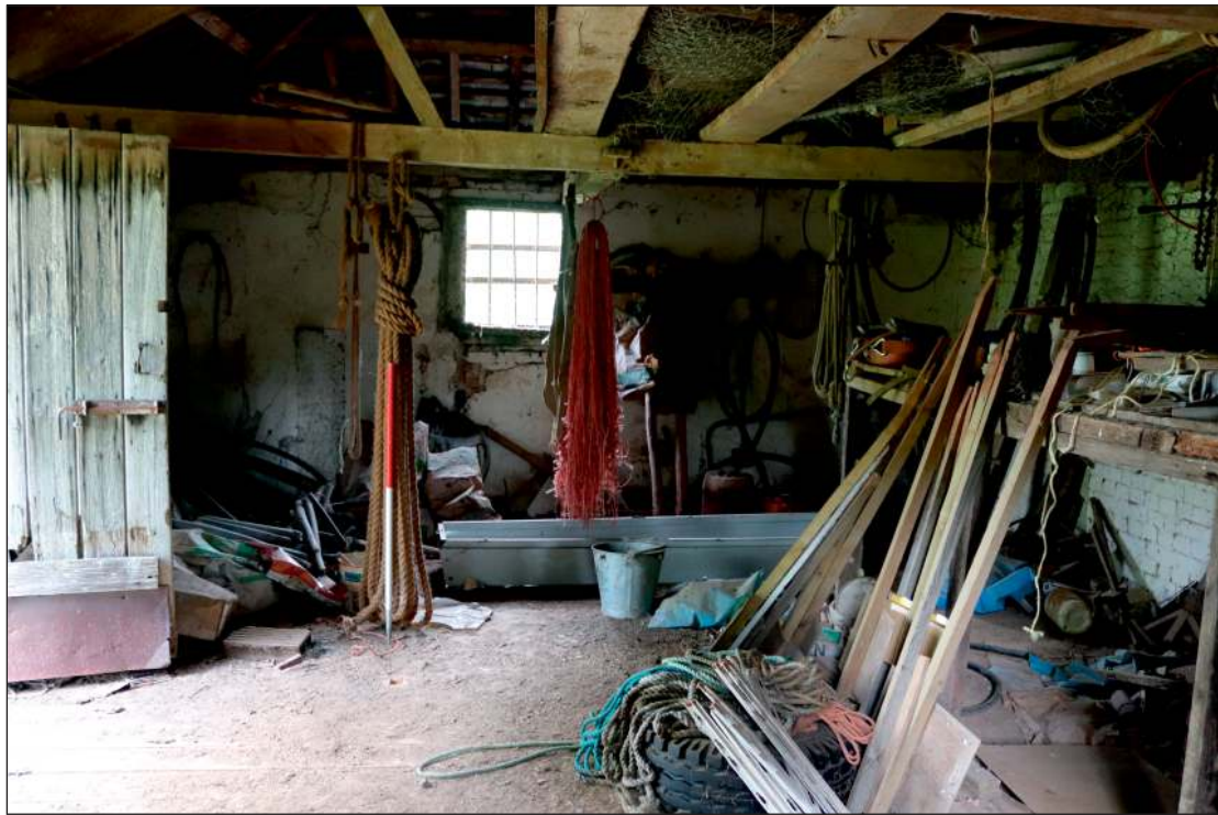
Plate 7: The interior of the first floor looking north, showing the original plastered timber frame of the north elevation and replacement brick east elevation to the right (1m scale)
