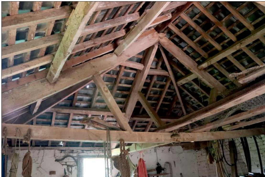
Plate 8: The north roof truss looking north-northeast
