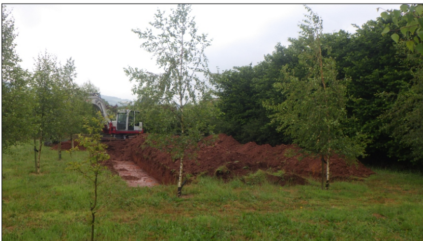
Plate 3: General working view of Trenches 5 and 6, looking southwest
