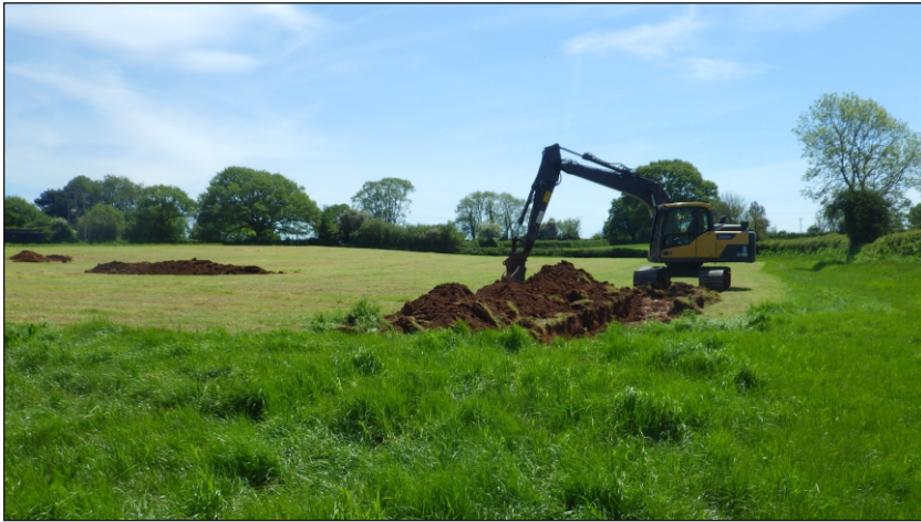
Plate 1: General working view with Trench 4 in foreground, looking southeast
