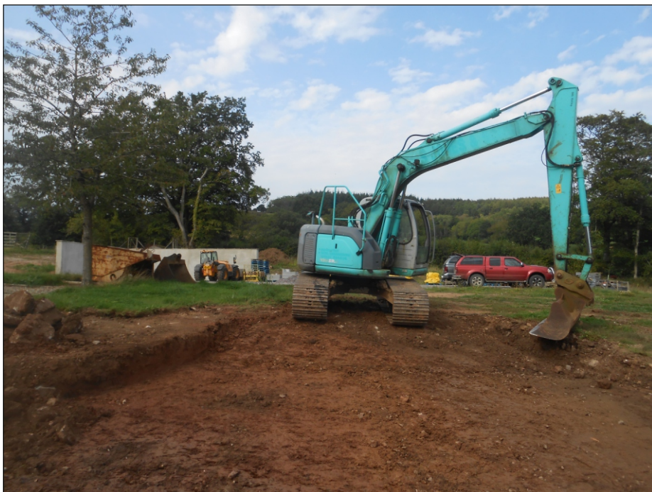
Plate 2: General view of groundworks in progress, looking west
