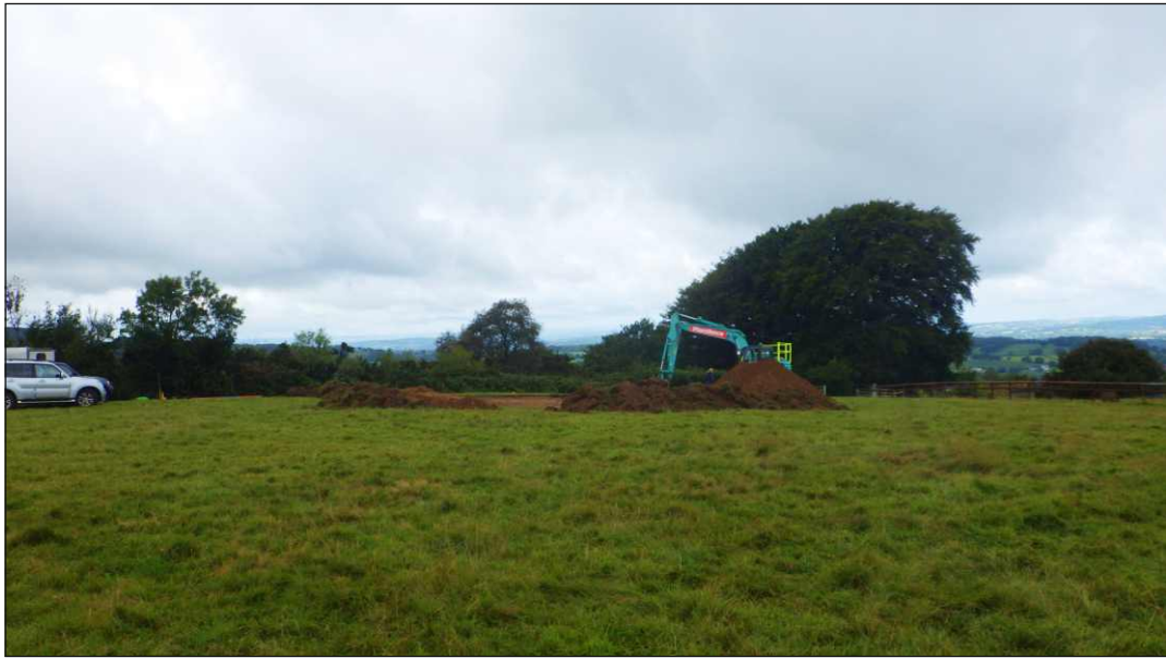
Plate 1: General view of site looking southwest
