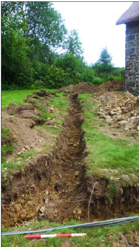
Plate 3: Showing excavated service trench, looking southeast (scale 0.4m)
