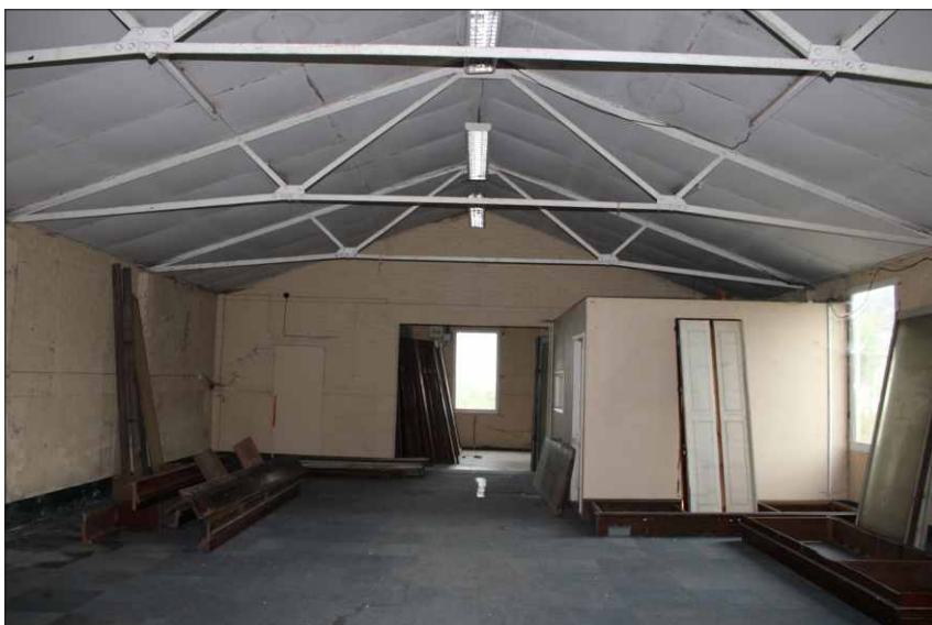
Plate 6: Central room of the institute and NAAFI, looking north (1m scale)
