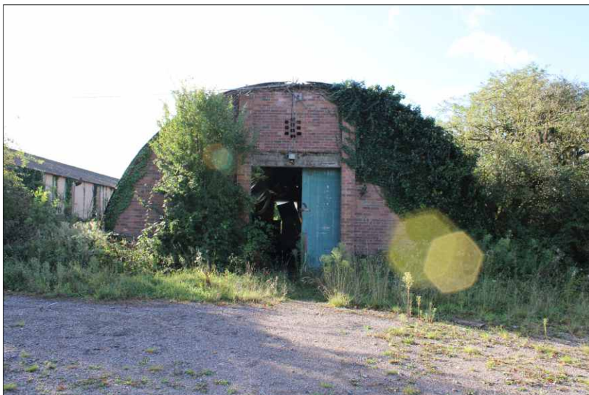
Plate 9: North elevation of the Romney hut, looking south (1m scale)
