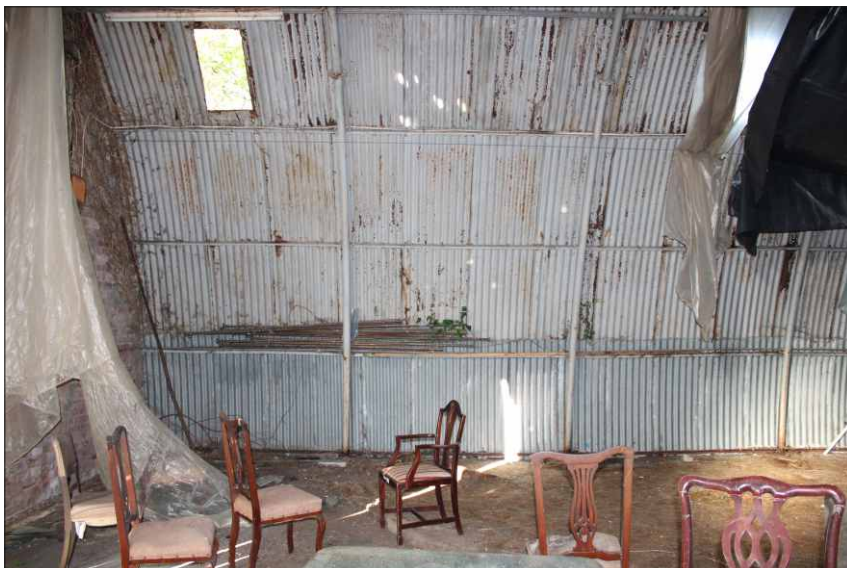
Plate 12: View of roof construction, looking west
