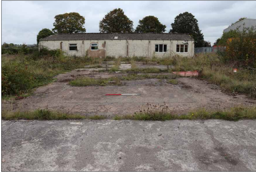
Plate 15: The concrete floor of the demolished central range, looking north (1m scale)
