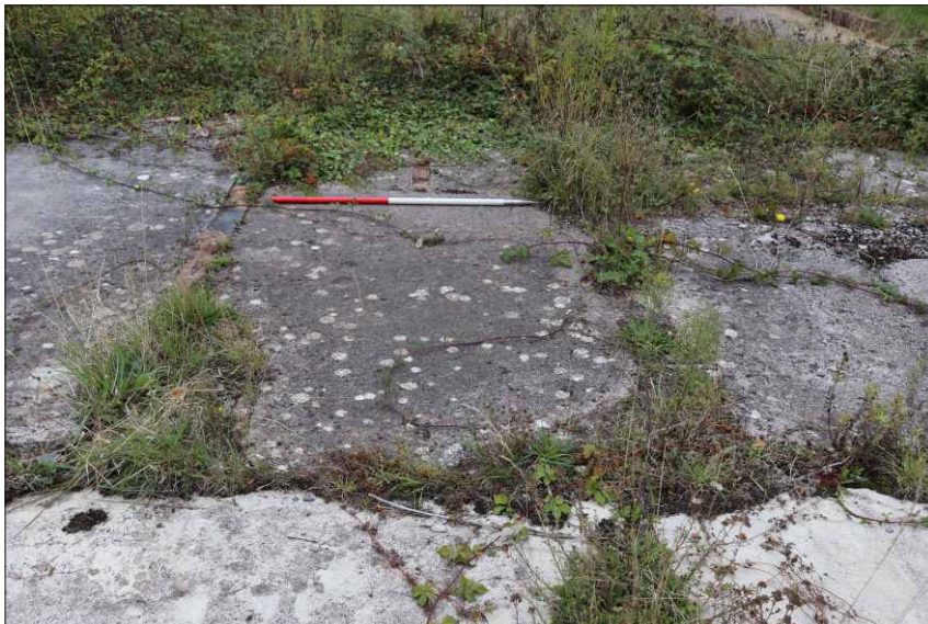
Plate 16: Brick scars in between concrete floors of the central range, looking west (1m scale)
