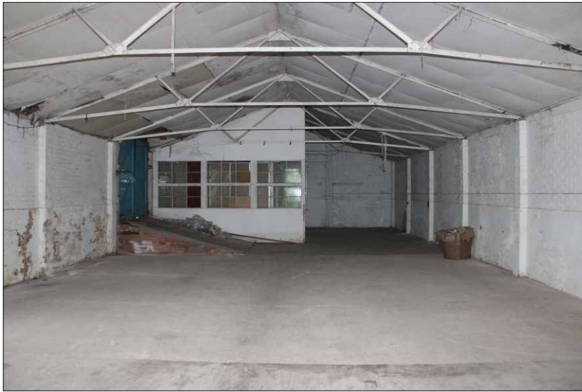
Plate 7: South room of the institute and NAAFI, looking south (1m scale)
