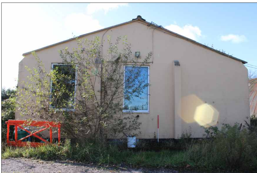
Plate 3: North elevation of the institute and NAAFI, looking south (1m scale)
