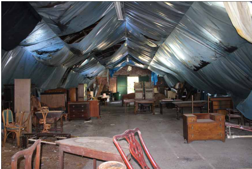
Plate 11: Internal view of the Romney hut, looking north
