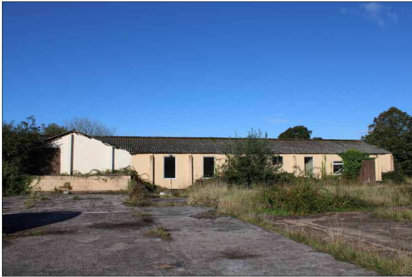
Plate 1: East elevation of the institute and NAAFI, looking west (1m scale)
