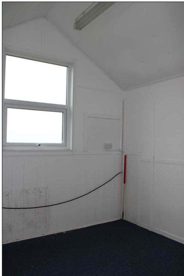
Plate 6: Internal view of room 2, looking north (1m scale)
