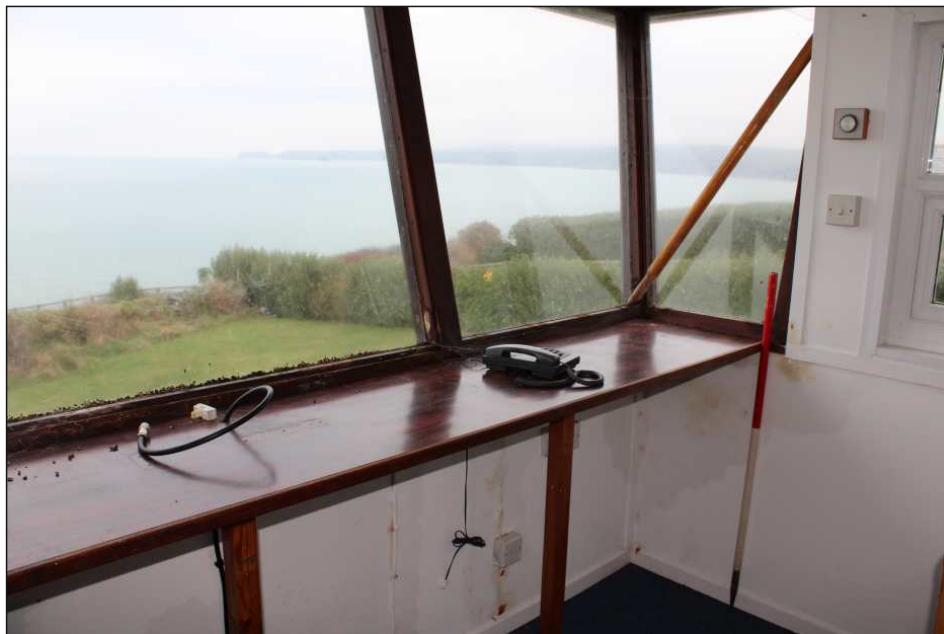
Plate 10: Internal view of room 1, looking northeast (1m scale)
