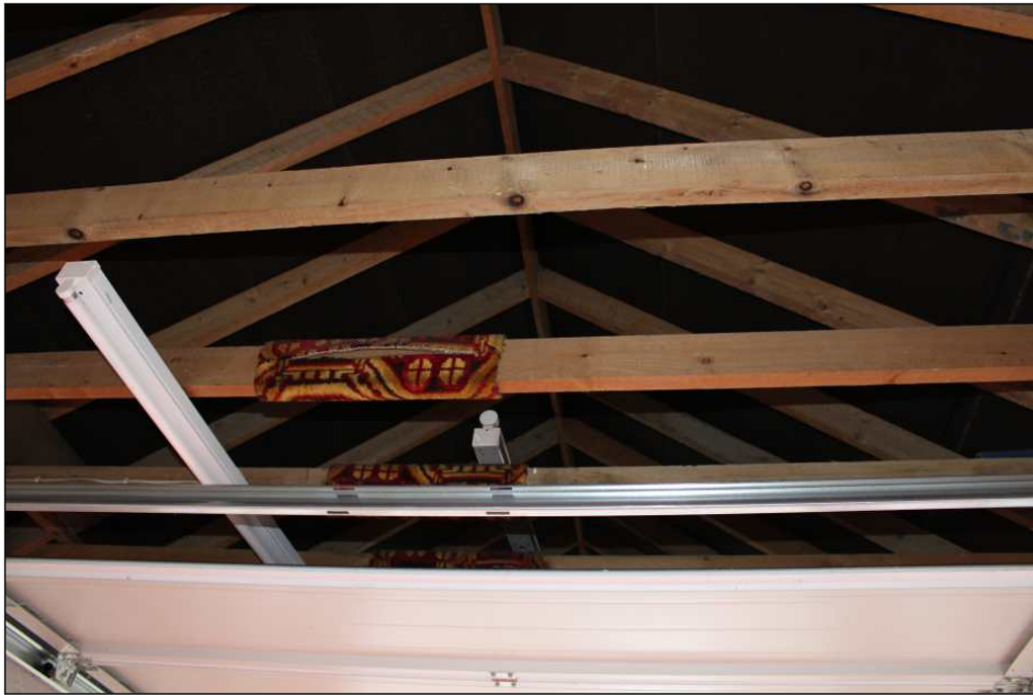
Plate 15: View of the roof structure of room 4, looking south
