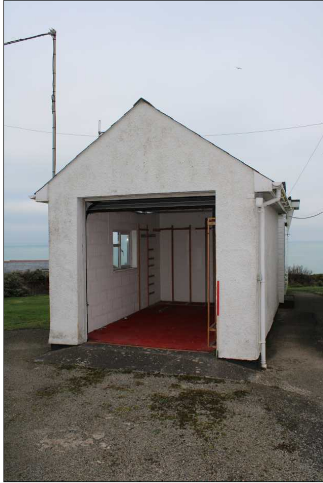
Plate 1: South elevation of the lookout, looking north (1m scale)
