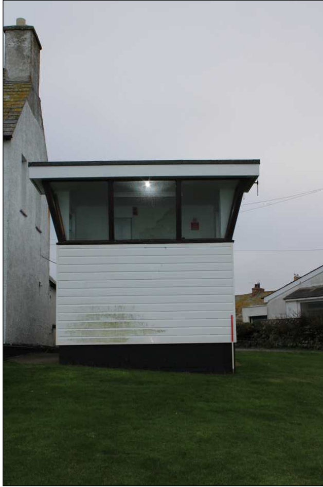
Plate 3: North elevation of the lookout, looking south (1m scale)
