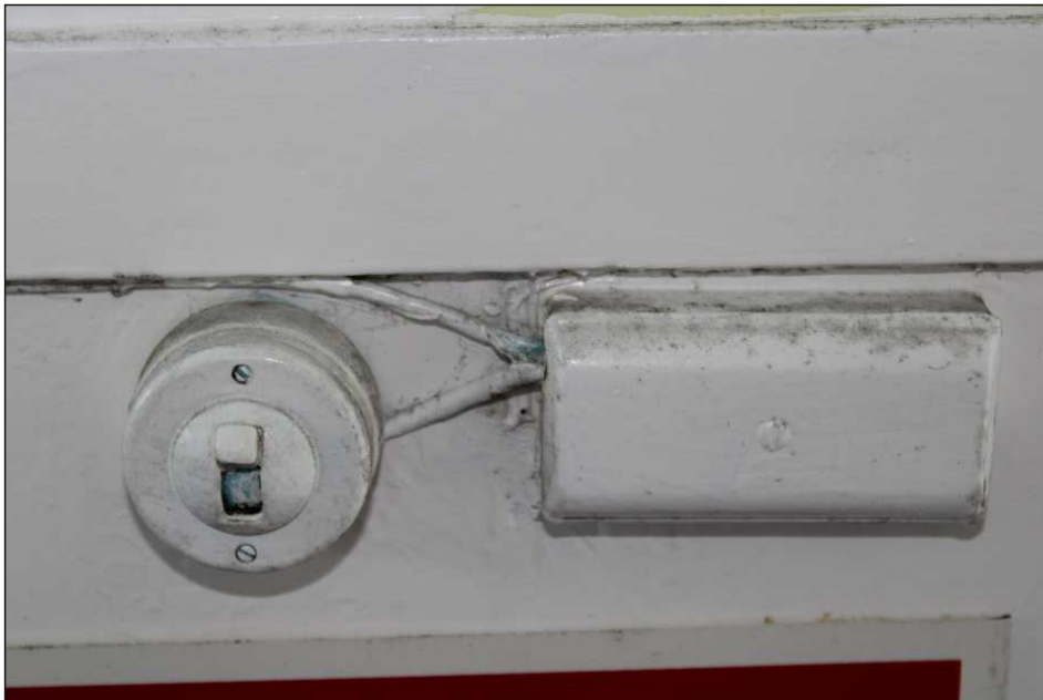
Plate 8: View of early-mid 20th century electrical fitting in room 2, looking east
