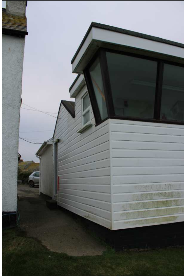
Plate 5: East elevation of the lookout, looking southwest (1m scale)
