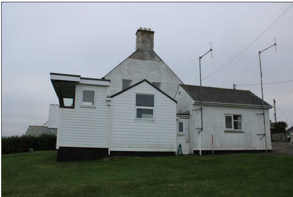
Plate 2: West elevation of the lookout, looking east (1m scale)
