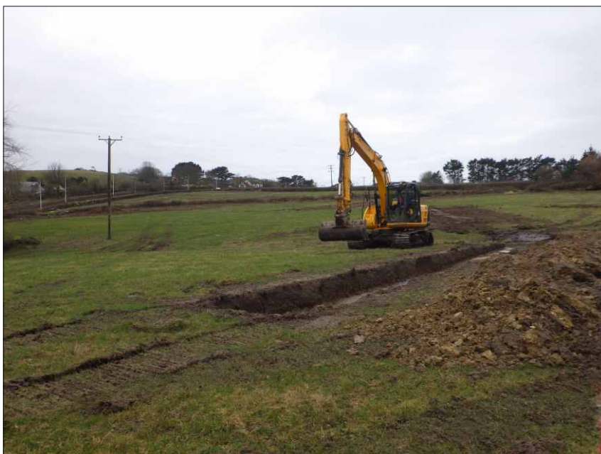
Plate 6: Trench 23, general view, looking west
