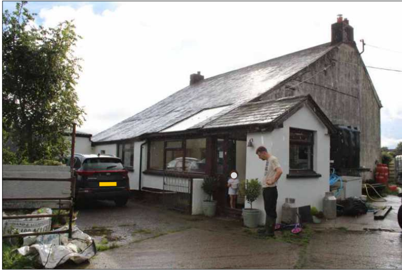
Plate 4: Northwest elevation, looking east
