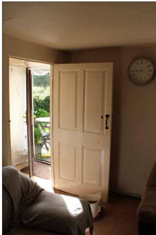
Plate 5: Four-panel door to reception room, looking east
