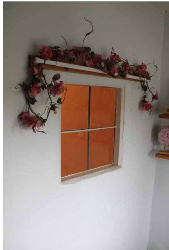
Plate 9: Window lighting staircase, looking north
