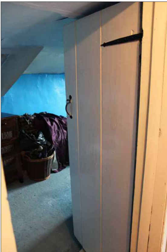
Plate 8: Plank and batten door to a bedroom on the first floor, looking north
