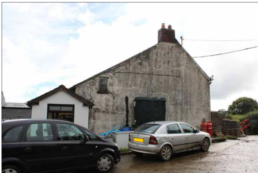
Plate 3: Southwest elevation, looking northeast
