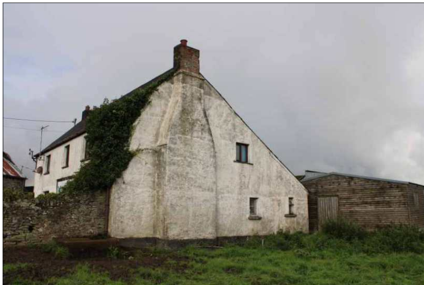
Plate 2: Northeast elevation, looking west
