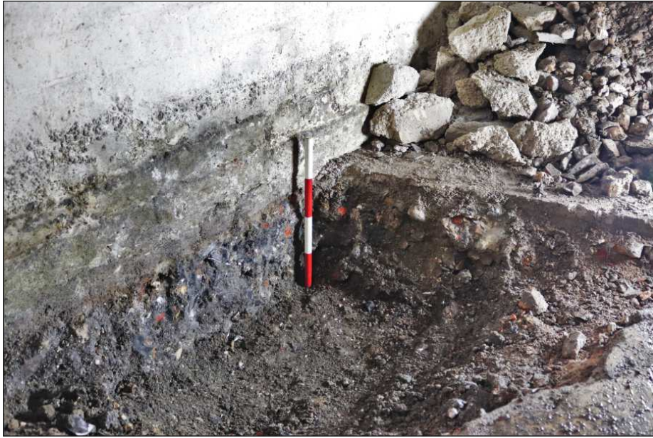
Plate 3: The northwest end of the service trench within the passage, looking north (0.40m scale)
