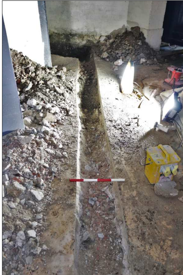
Plate 1: The service trench, looking northwest (0.40m scale)
