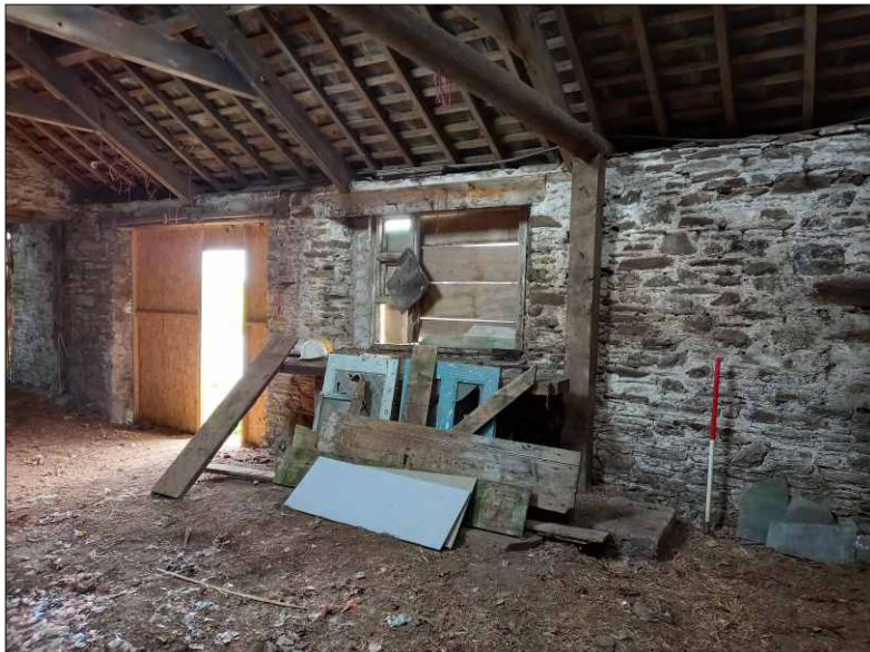
Plate 2: Internal view of south wall, showing the narrowed window, looking east (1m scale)
