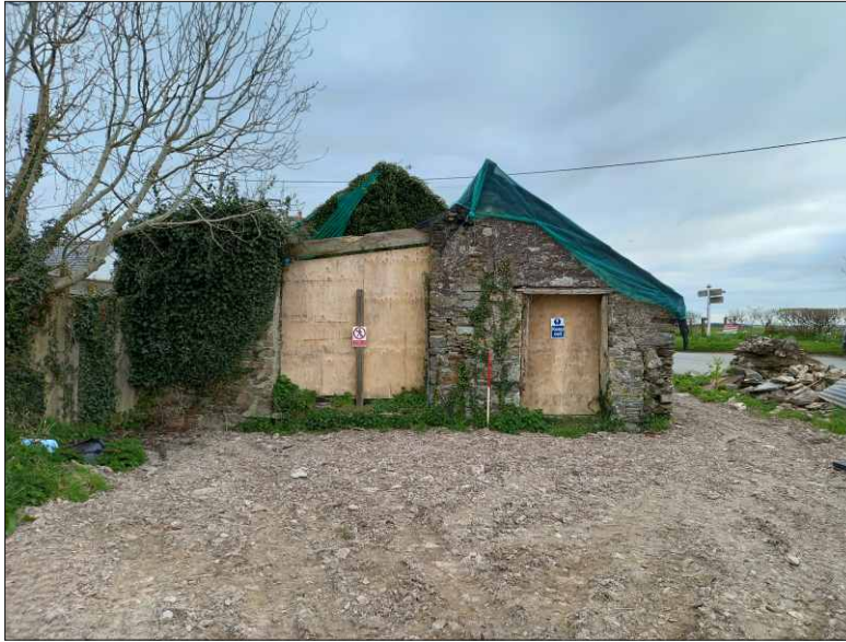
Plate 7: West elevation of the extension, looking northeast (1m scale)
