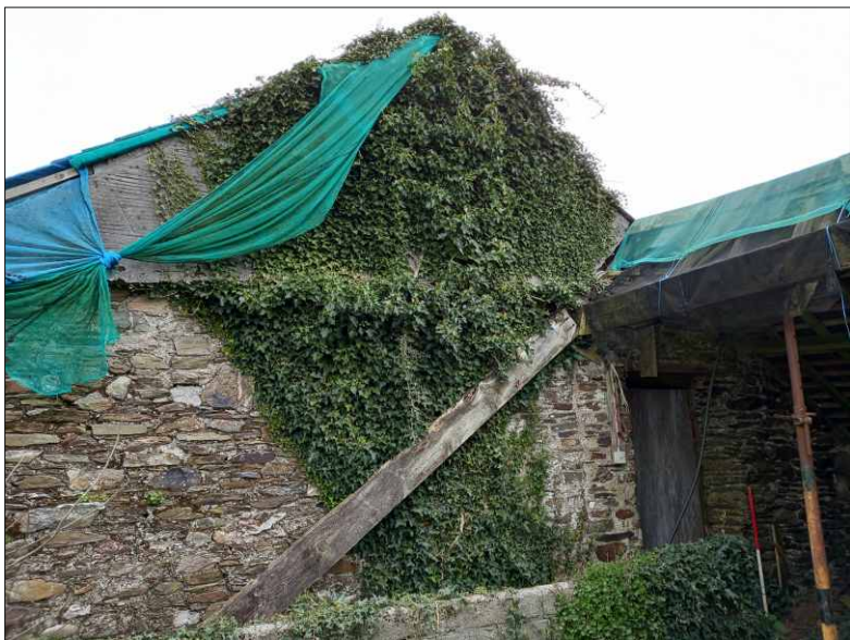
Plate 6: West elevation, looking east (1m scale)
