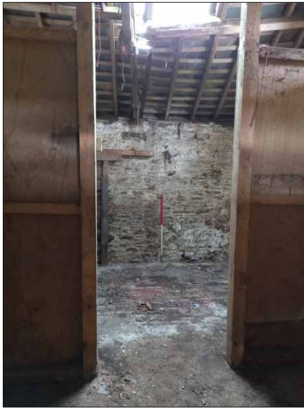
Plate 10: East room, looking northwest (1m scale)
