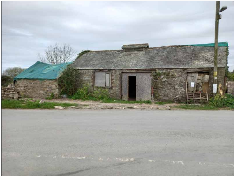
Plate 1: South elevation, looking northwest (1m scale)
