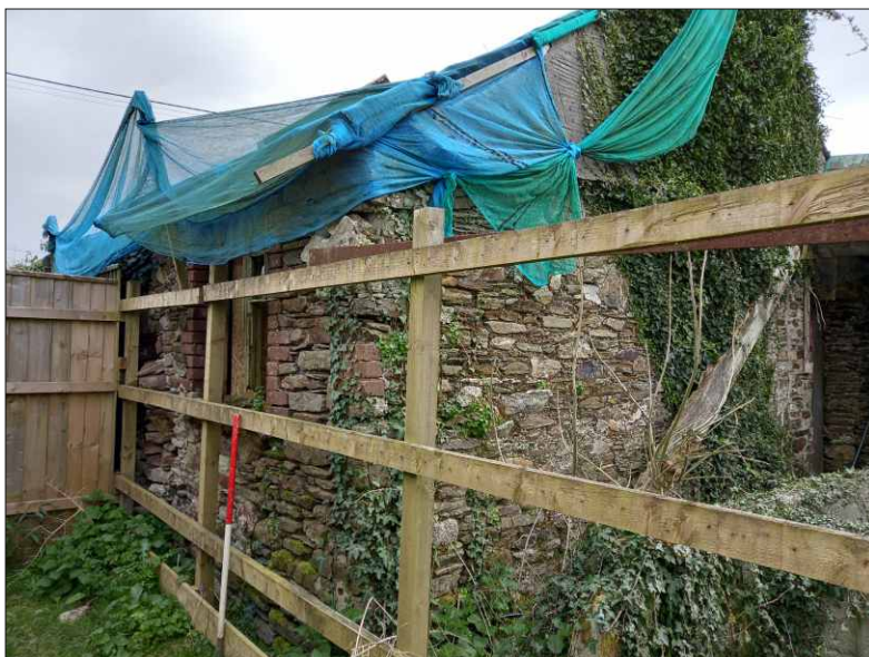
Plate 3: Northwest corner of the building, looking east (1m scale)
