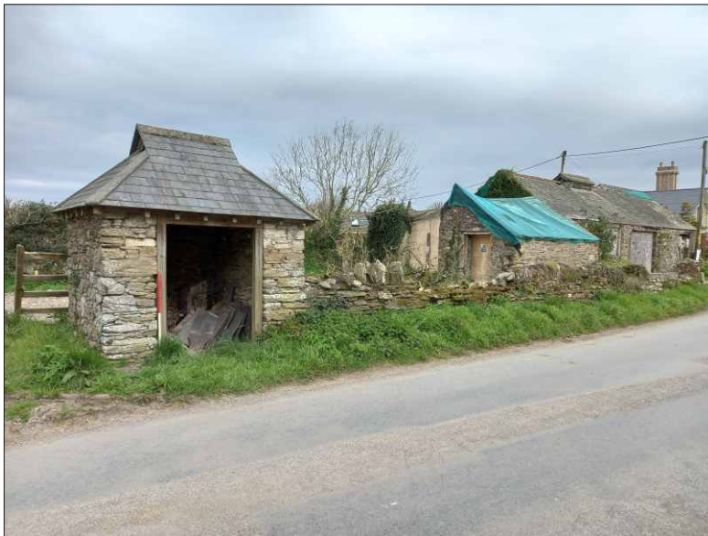
Plate 8: View of pump house and boundary wall, looking north (1m scale)
