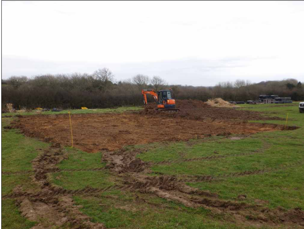
Plate 1: General view of the site, work in progress, looking north
