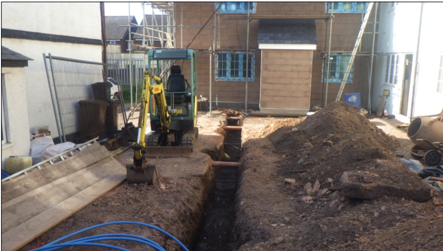
Plate 2: General view of trial trench, looking south
