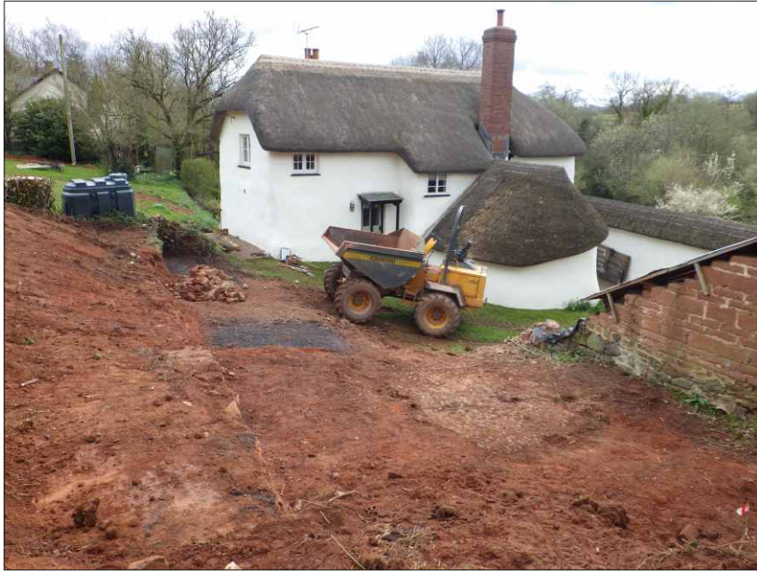
Plate 1: General view of the site, looking south
