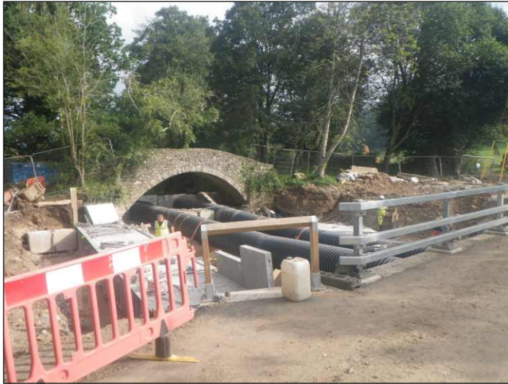
Plate 1: View of Beckford Bridge. Looking north
