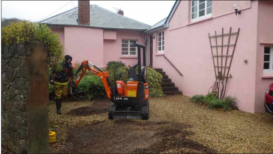
Plate 1: General view of the working area, looking southwest
