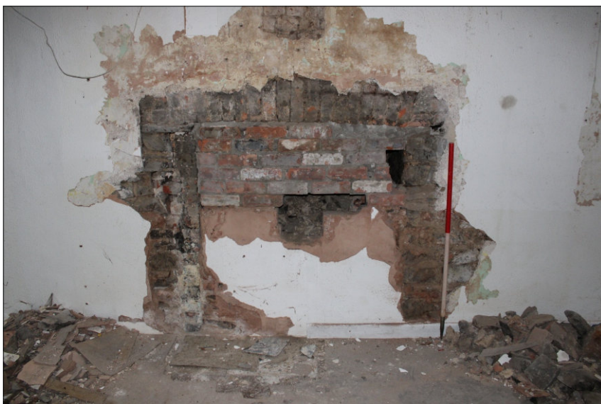
Plate 6: Blocked fireplace in the west wall, looking northwest (1m scale)
