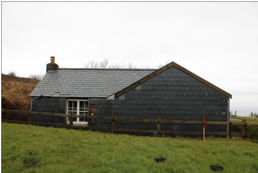
Plate 2: South elevation, looking northeast (1m scale)
