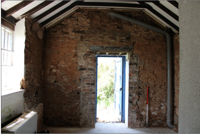
Plate 16: West wall of south extension, showing doorway cutting through former fireplace, looking northwest (1m scale)
