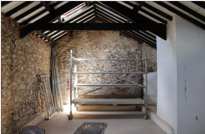
Plate 11: North and west walls showing projecting plinth, wall scar to left, and blocked fireplace with chimney stack, looking northeast (1m scale)
