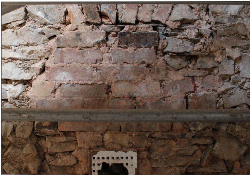
Plate 12: Close-up view of blocked fireplace in the north wall, looking northeast
