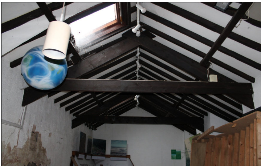
Plate 5: Roof structure, looking northeast
