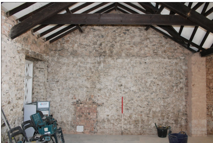
Plate 15: South wall with blocked fireplace, looking southwest (1m scale)
