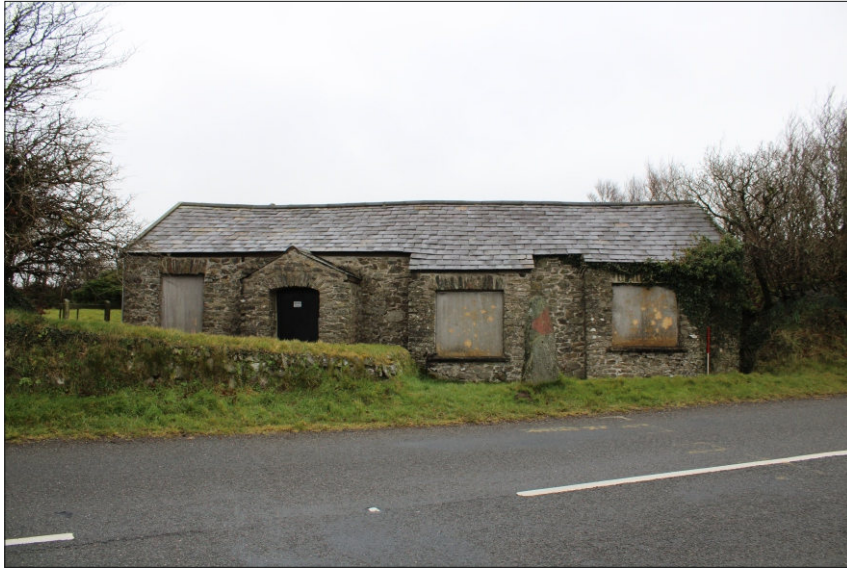
Plate 1: Main façade, looking northwest (1m scale)
