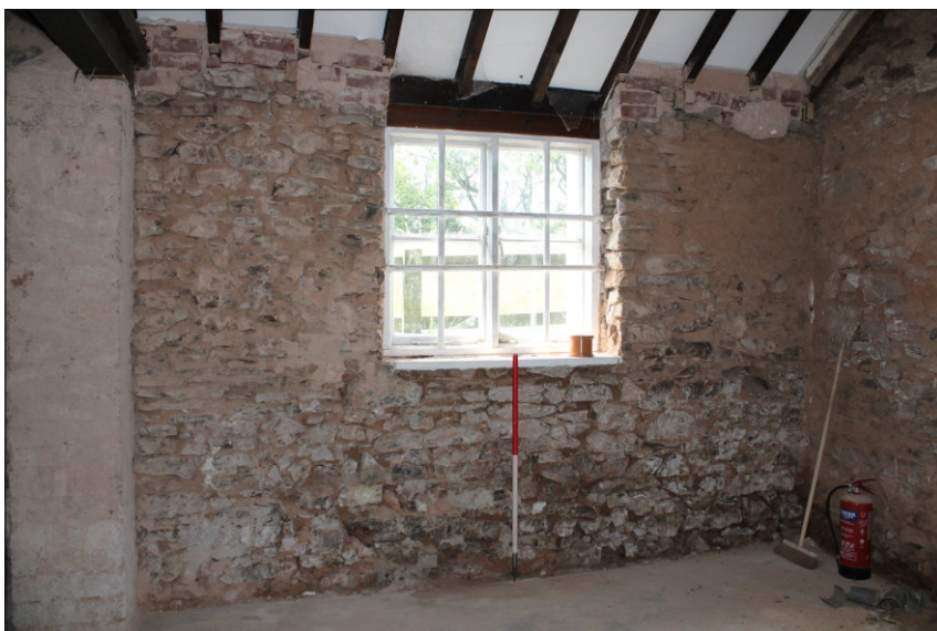
Plate 18: South wall of south extension, looking southwest (1m scale)
