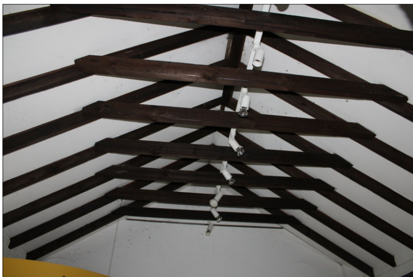
Plate 9: Roof structure of south extension, looking northwest
