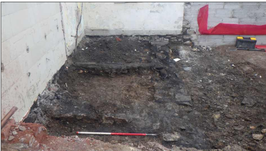
Plate 4: 19th century foundations S135, S137 and S138, view to northwest (scale 1m)
