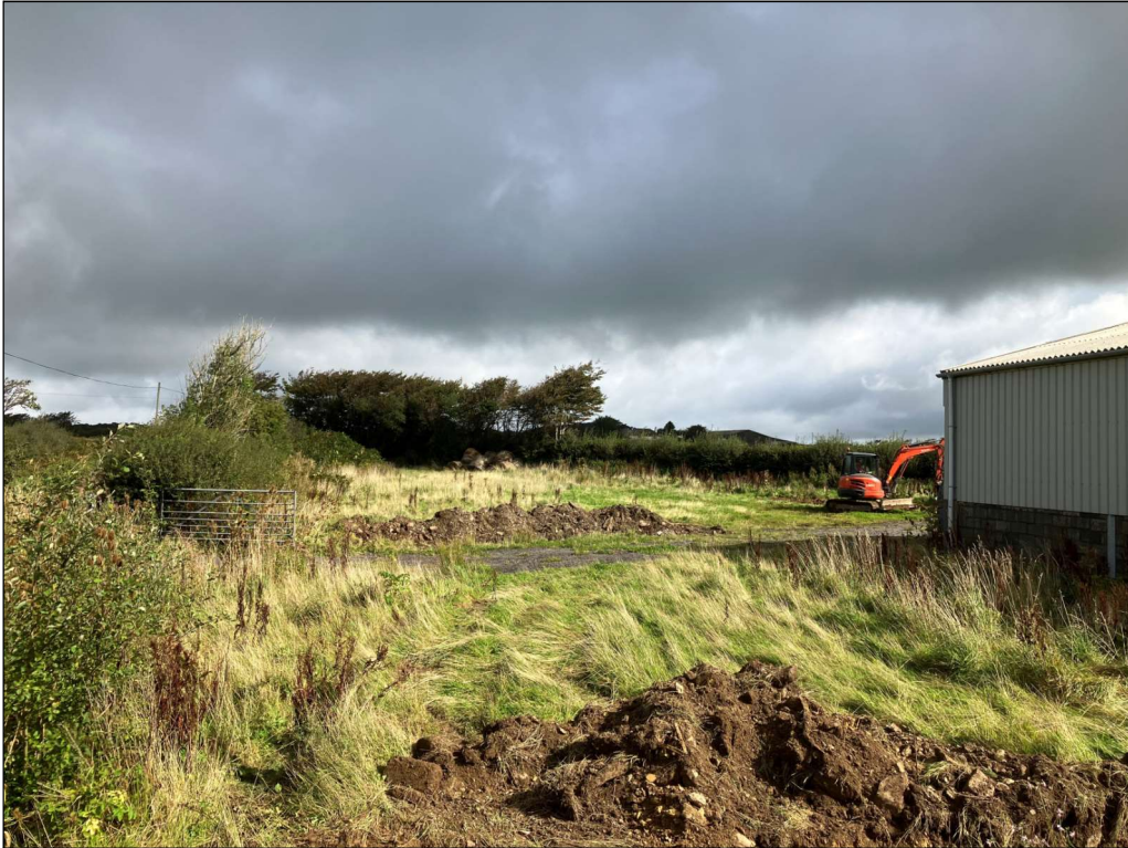
Plate 1: General working view of site, looking north towards Scheduled barrow with Trench 3 in background
