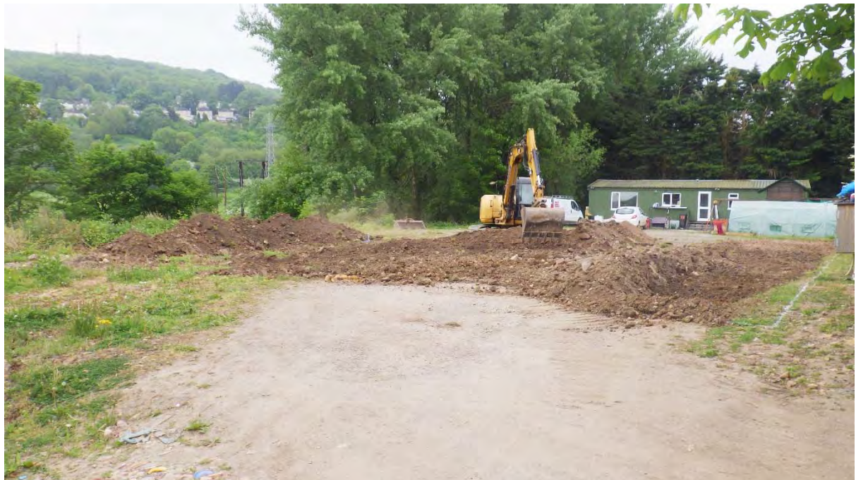
Plate 2: View of site (from north)
