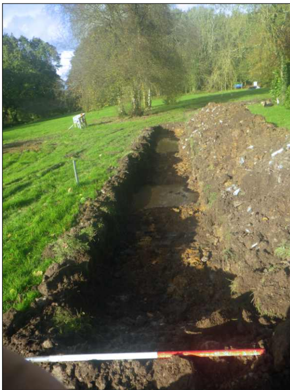
Plate 2: Trench 1, view to north (scale 1m)
