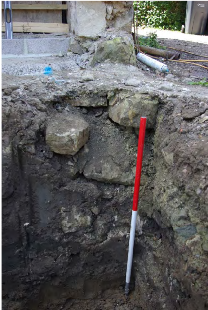
Plate 3: Foundations of demolished barn (wall of cottage in background)
