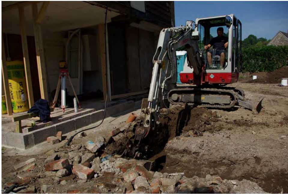
Plate 1: General view of groundworks
