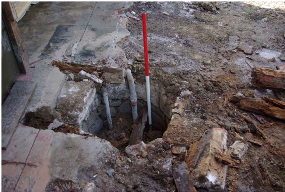
Plate 2: Well prior to foundation trench excavation
