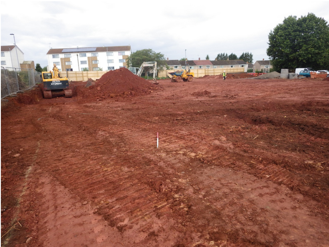
Plate 2: General view of site following topsoil strip, facing west. Scale 1m
