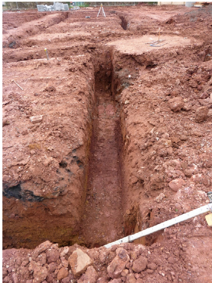
Plate 4: General view of foundation trenches, facing east
