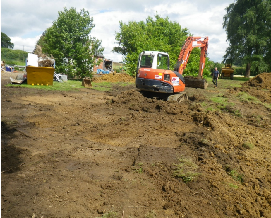
Plate 1: General view of groundworks
