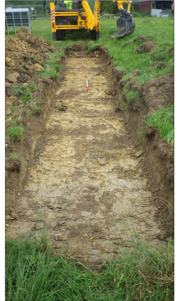
Plate 6: View along Trench 6 from the southwest (Scale 2m)
