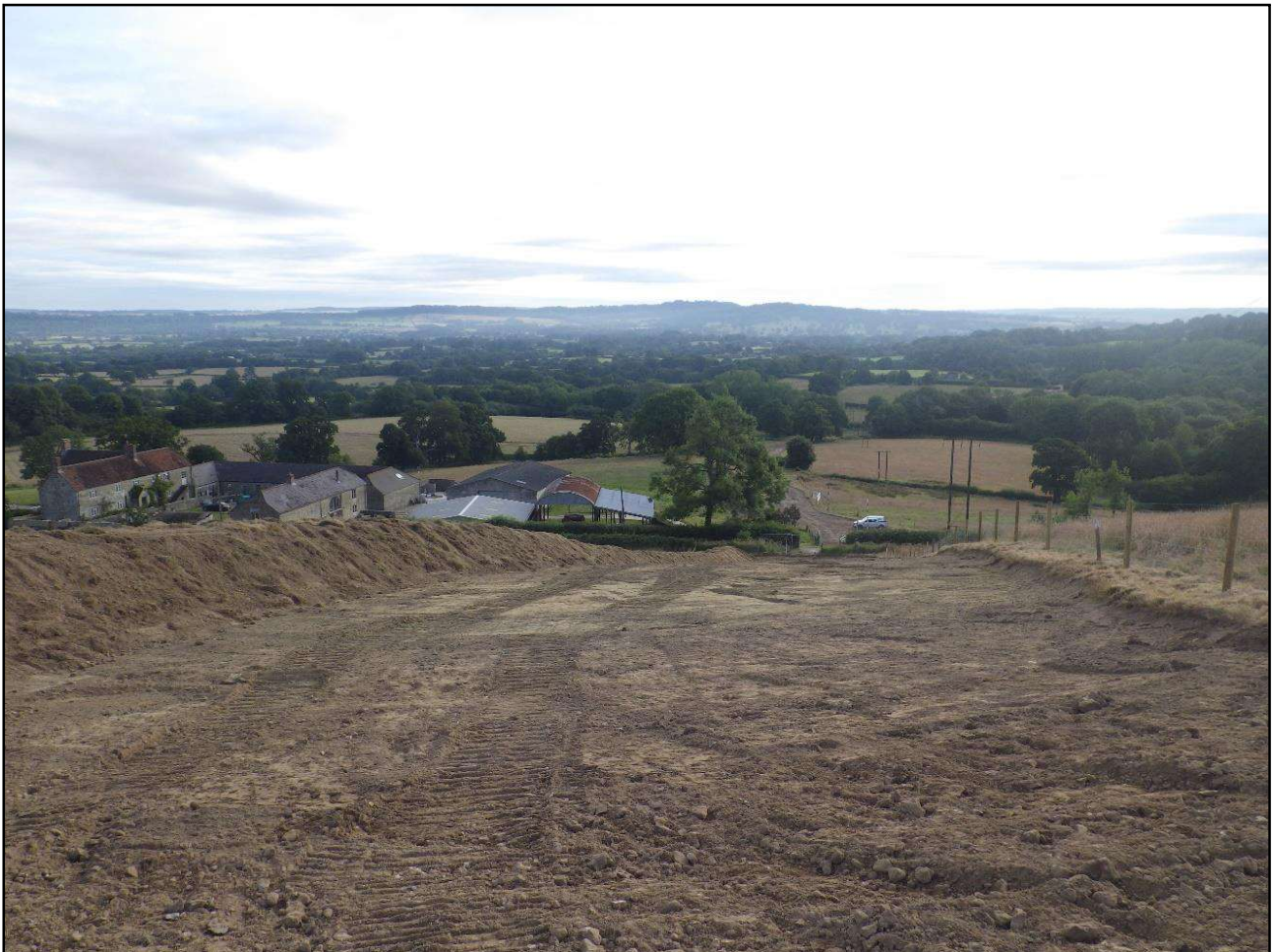
Plate 2: Completed easement strip. View from the south-west
