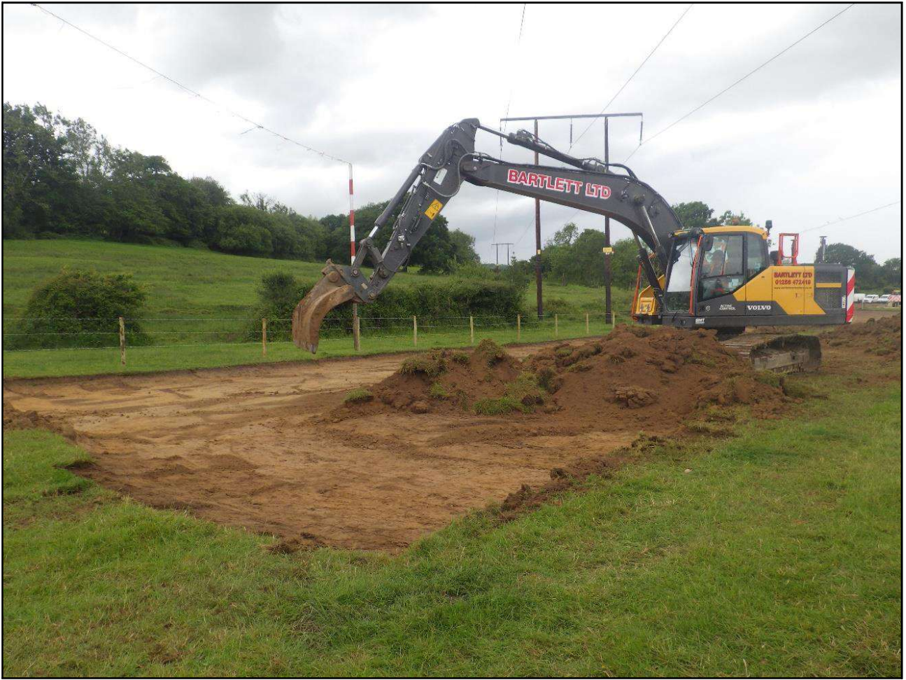
Plate 1: Working view of easement strip with earthworks in the background
