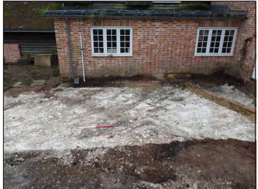
Plate 4: South facing natural geology in development area (scale 1m)
