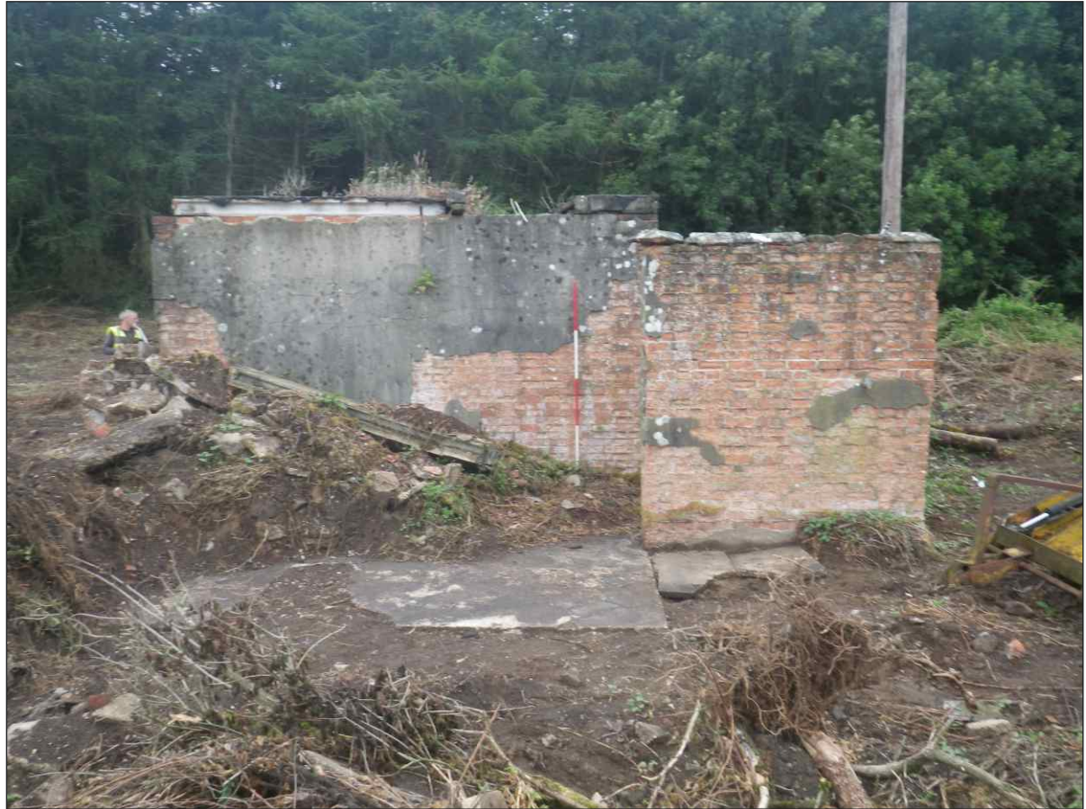
Plate 2: Southeast facing elevation (scale 2m)
