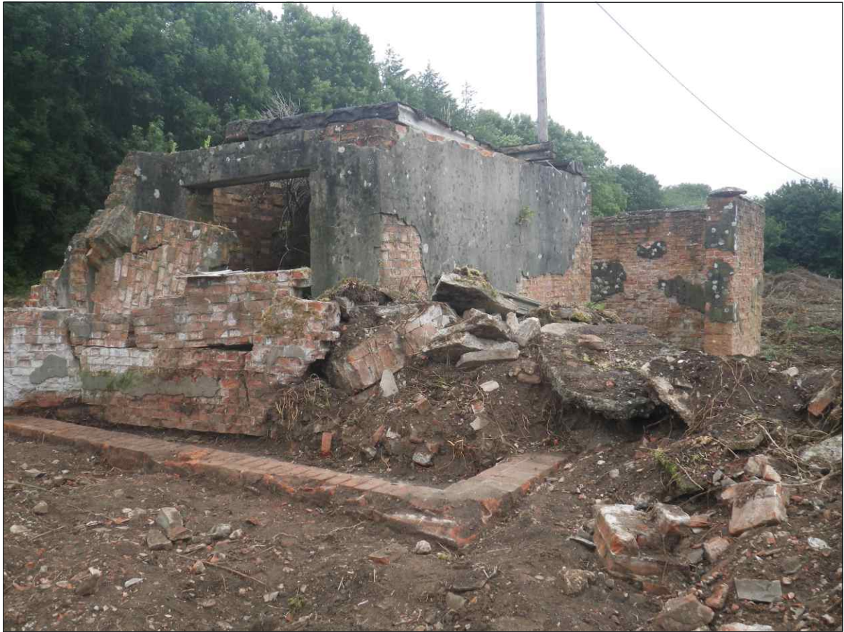
Plate 5: General view of the building from the south
