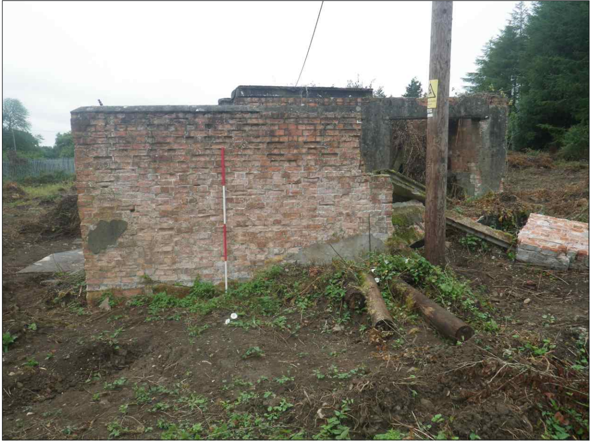
Plate 1: Northeast facing elevation (scale 2m)
