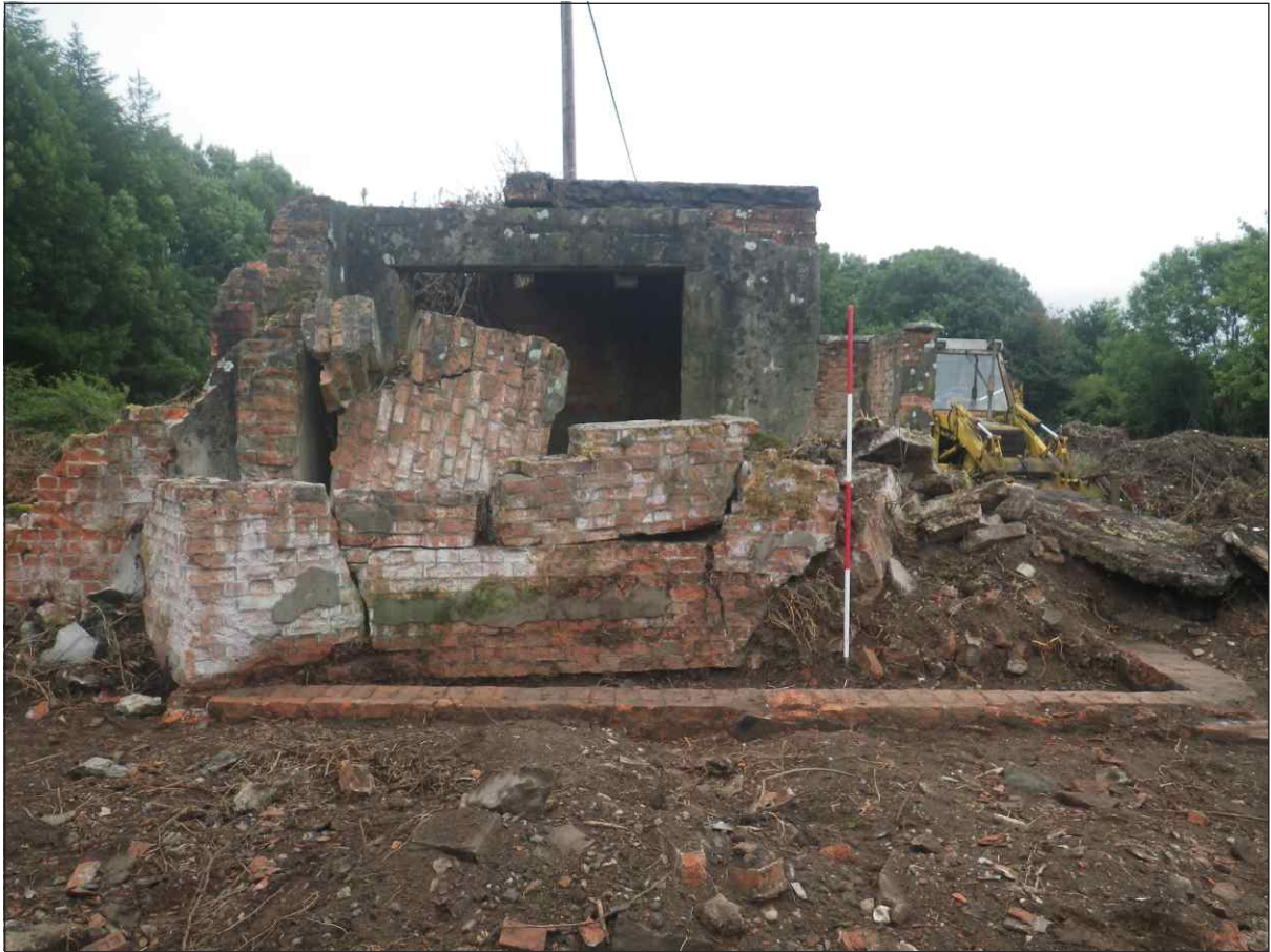
Plate 3: Southwest facing elevation (scale 2m)
