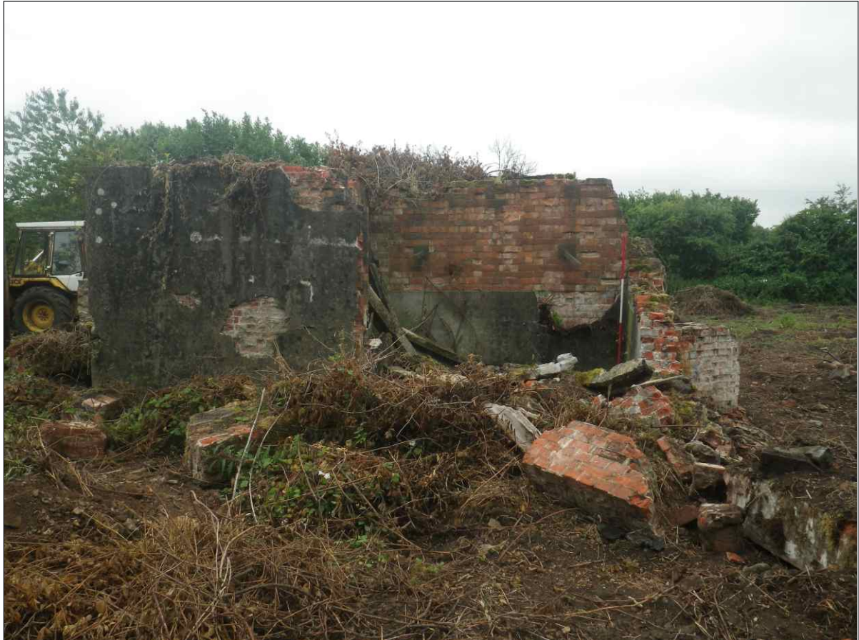
Plate 4: Northwest facing elevation (scale 2m)
