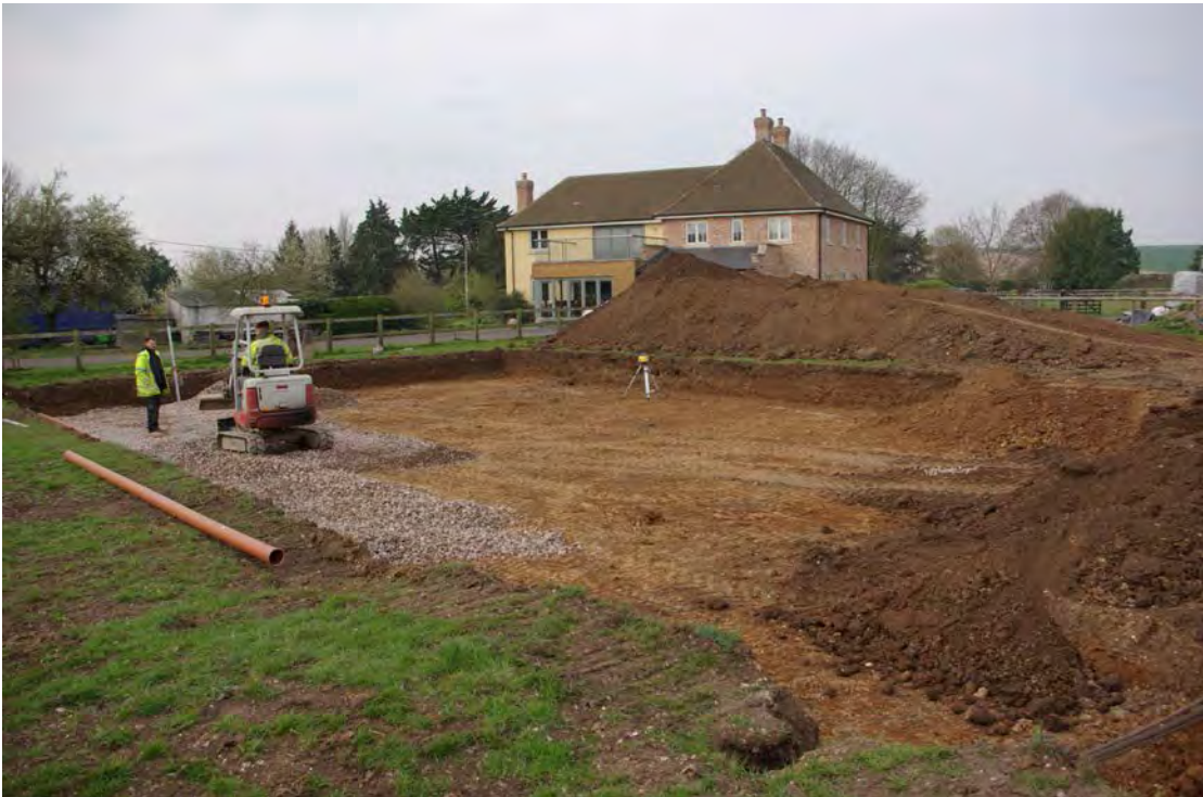
Plate 2: General view of groundworks
