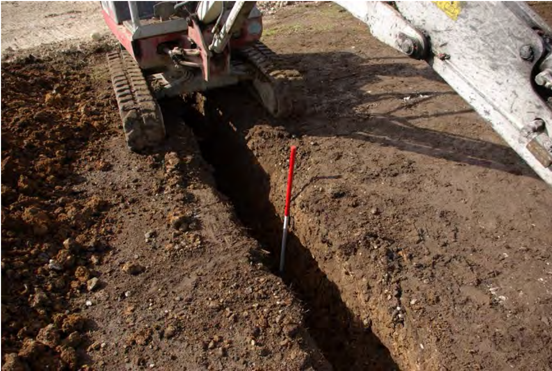
Plate 4: Pipe trench linking soak-away with treatment plant
