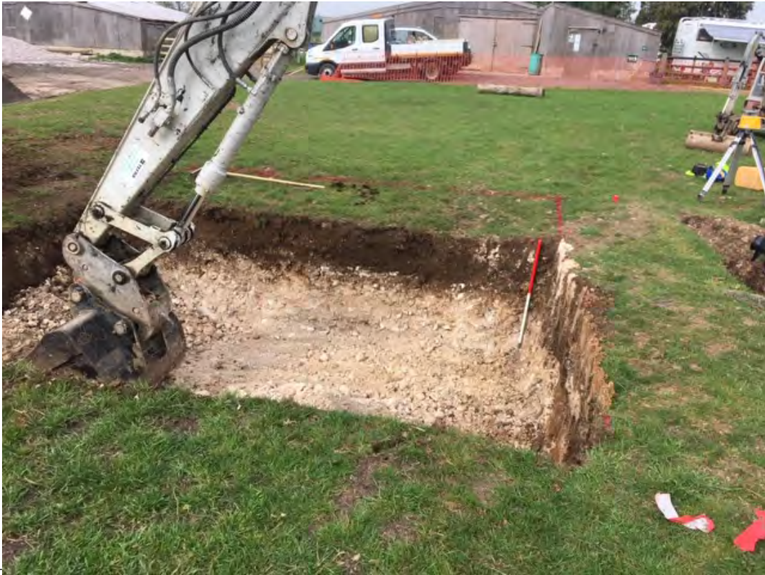
Plate 3: Excavation of sewage treatment plant area
