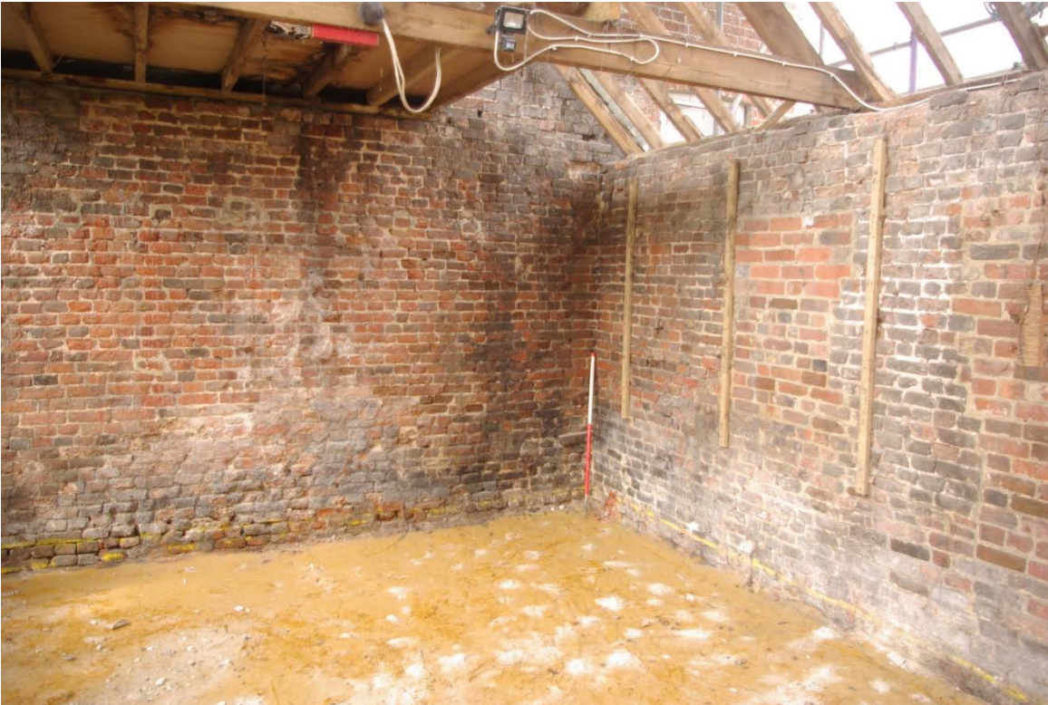
Plate 3: Interior of building
