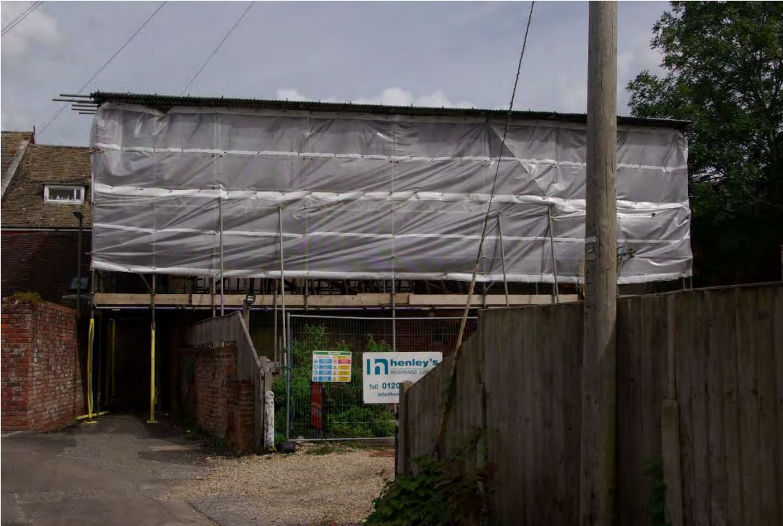
Plate 1: General view of building showing protective screening
