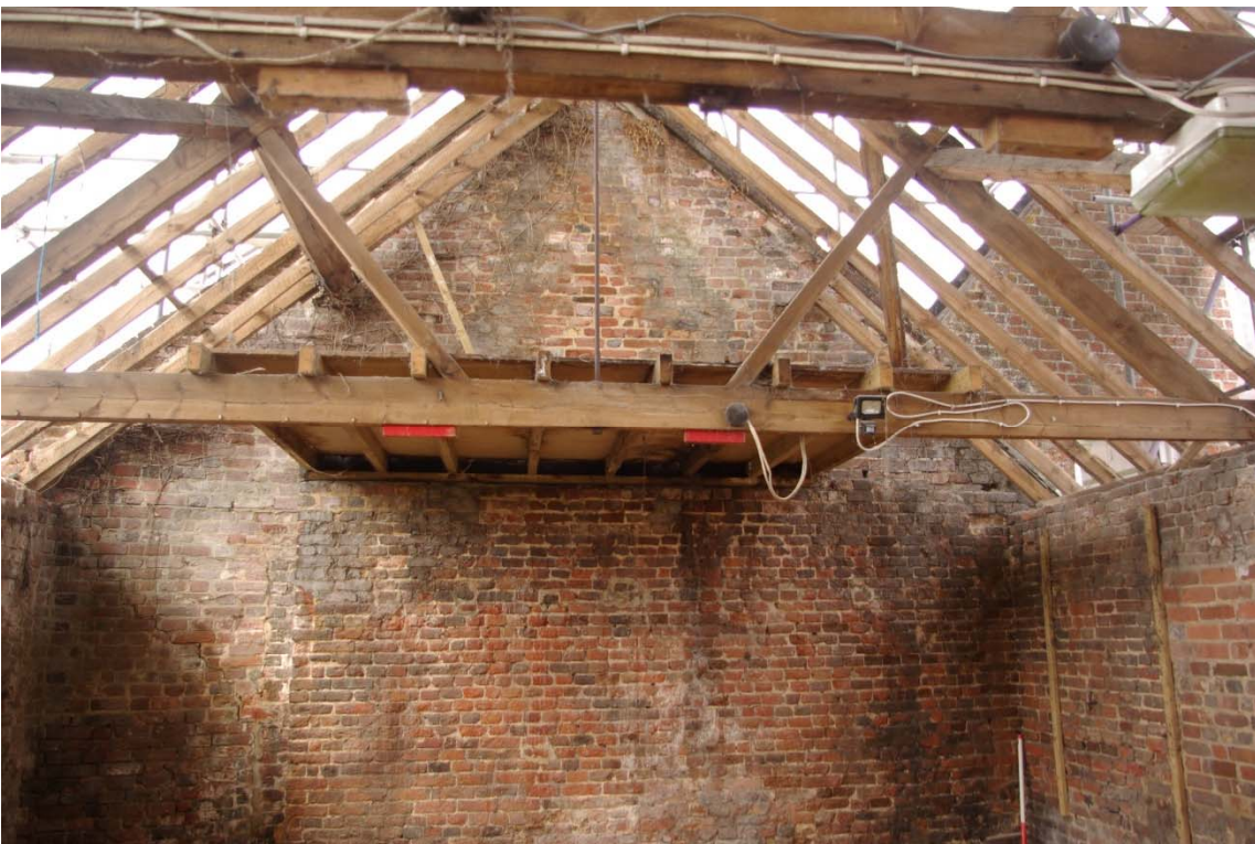
Plate 2: General view of interior and roof timbers
