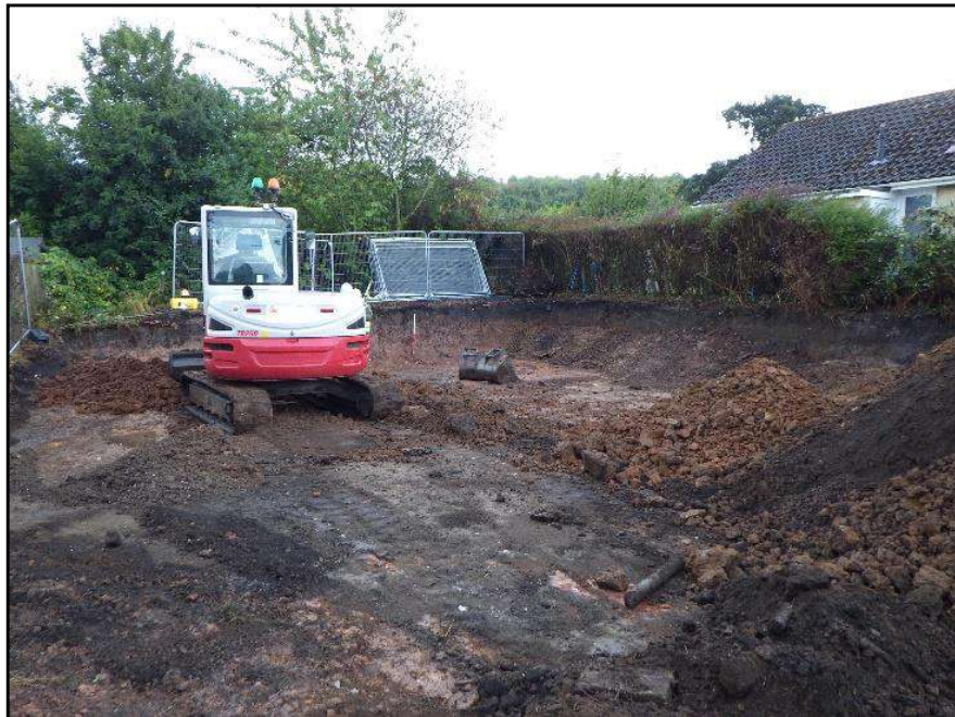
Plate 3: General view of groundworks
