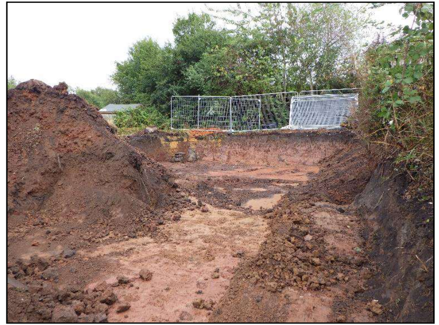
Plate 2: Reduced levels at rear of site
