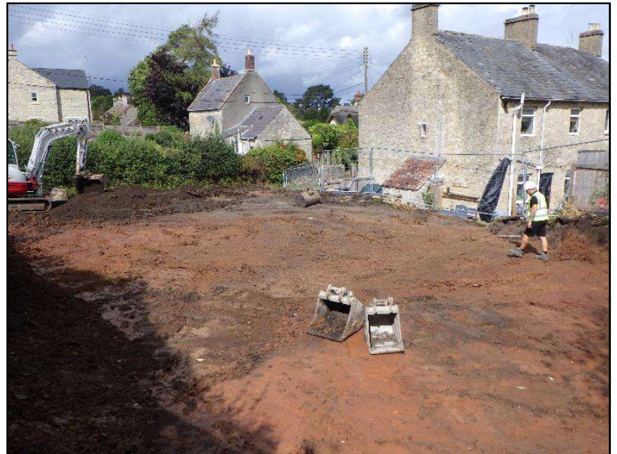
Plate 4: General view at completion of groundworks
