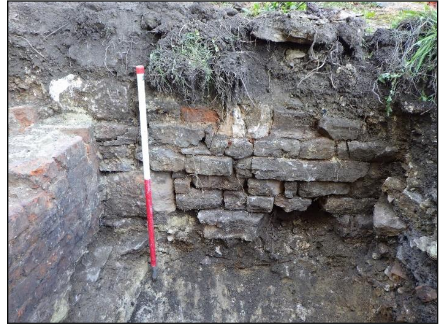
Plate 2: South facing section showing wall S103 (scale 1m)
