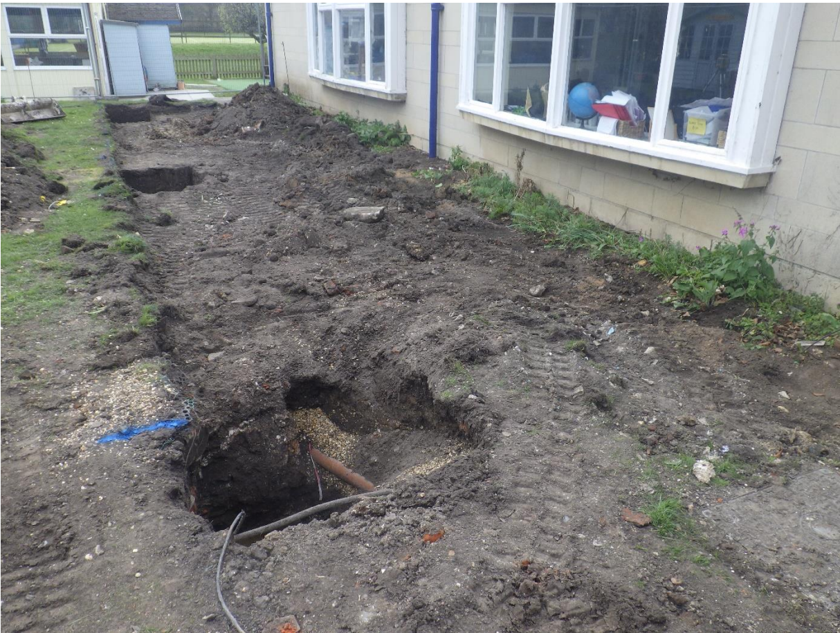
Plate 1: View of site following the removal of topsoil, with post-pads 1 – 3 visible.
