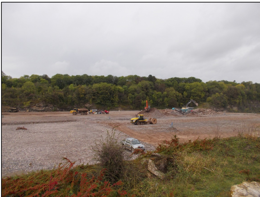
Plate 1: The disused Barnhill Quarry during backfilling operations prior to the development
