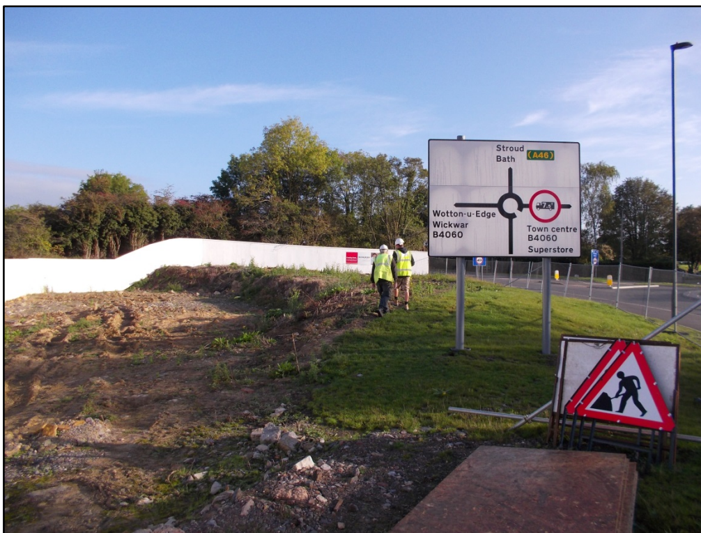
Plate 2: Area north of Drovers Way prior to excavation
