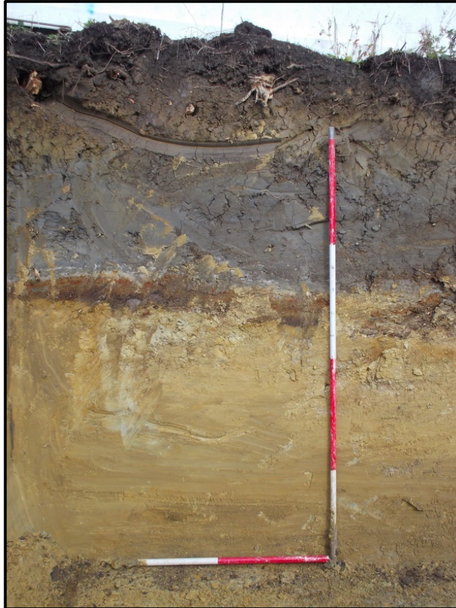
Plate 5: North-facing section at northern extent of area north of Drovers Way showing exposed soil sequence during excavation of foundation trenches. Scale 2m/1m
