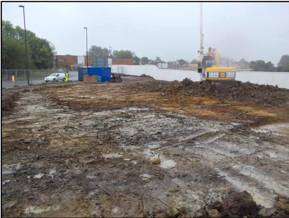
Plate 4: Partial reduced level dig showing the mixed overburden fills
