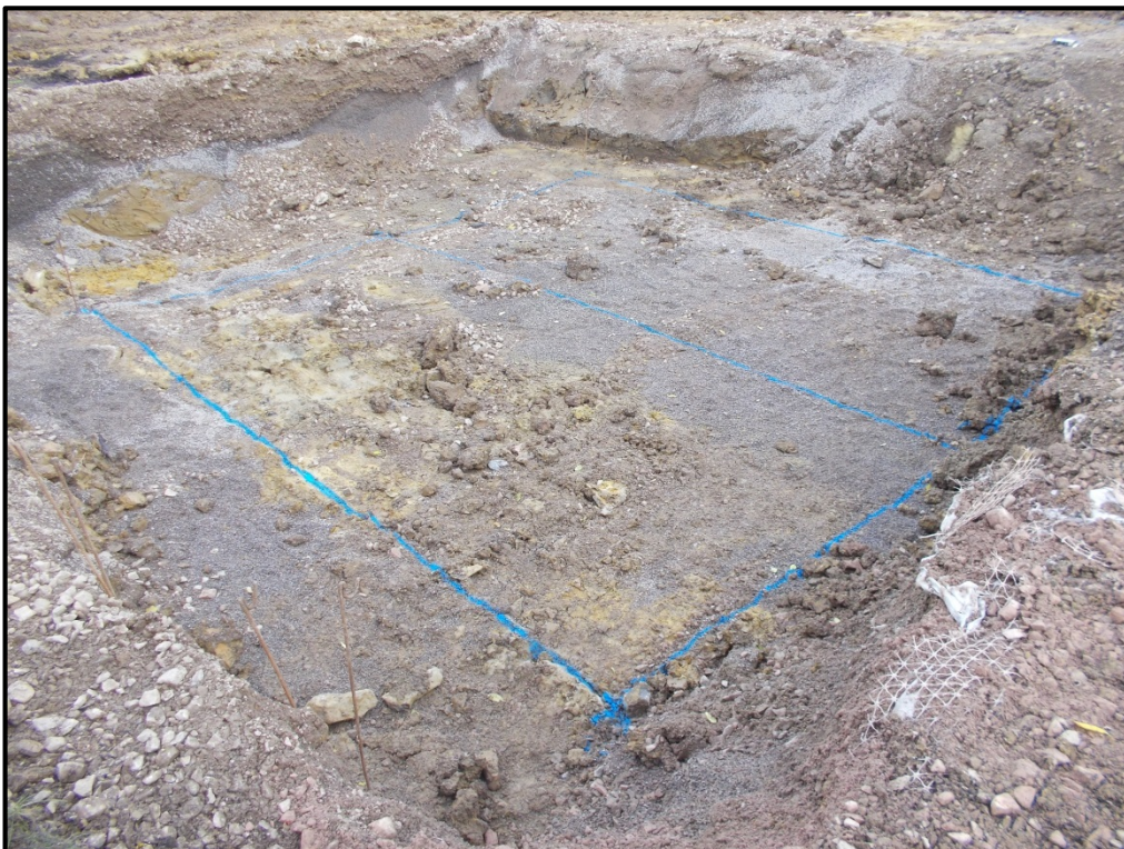
Plate 10: The exposed ground after reduced level dig
