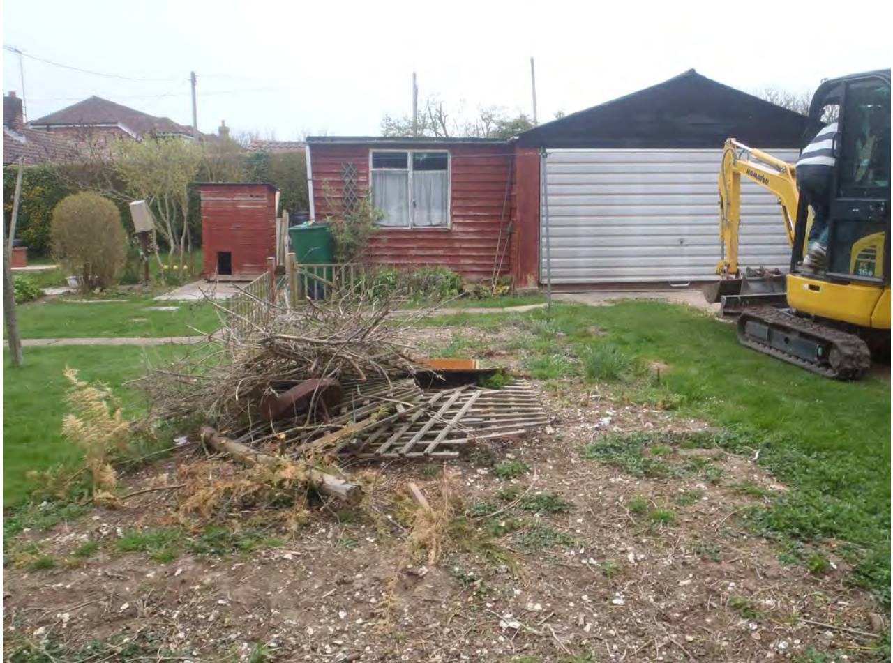
Plate 1: General view from the south prior to commencement of works
