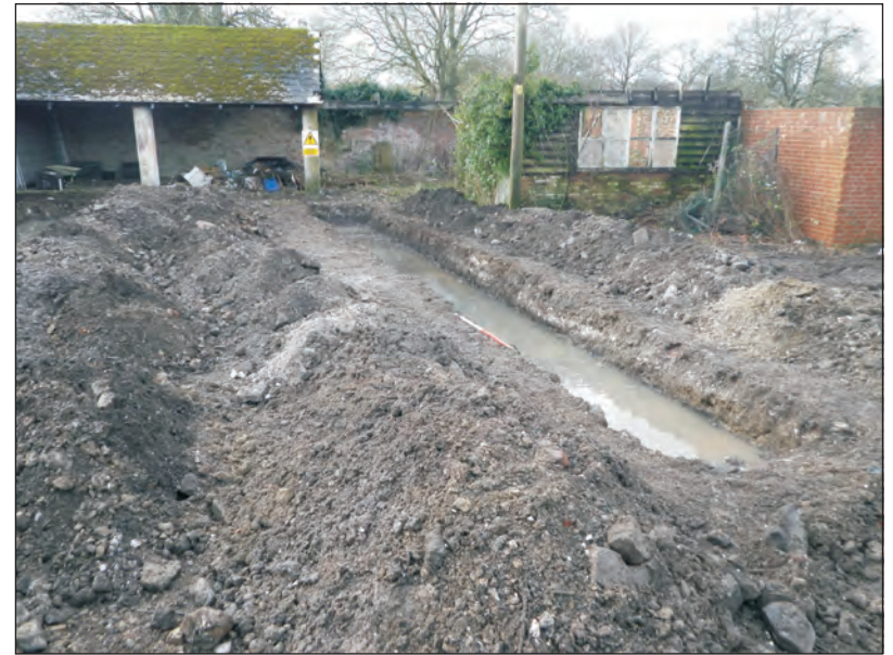
Plate 2: Trench 2, view from the north (scale 1m)
