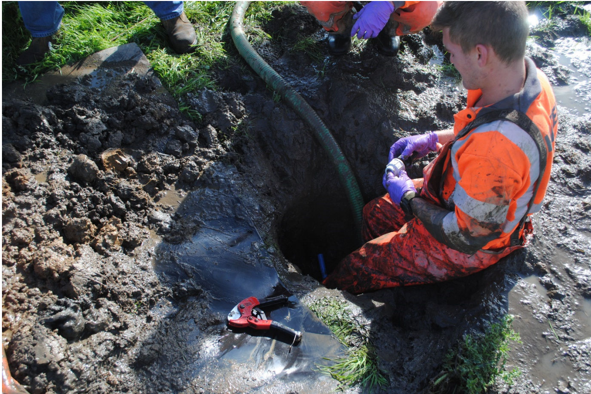
Plate 3: Detail of pipe repair works in progress. View from west
