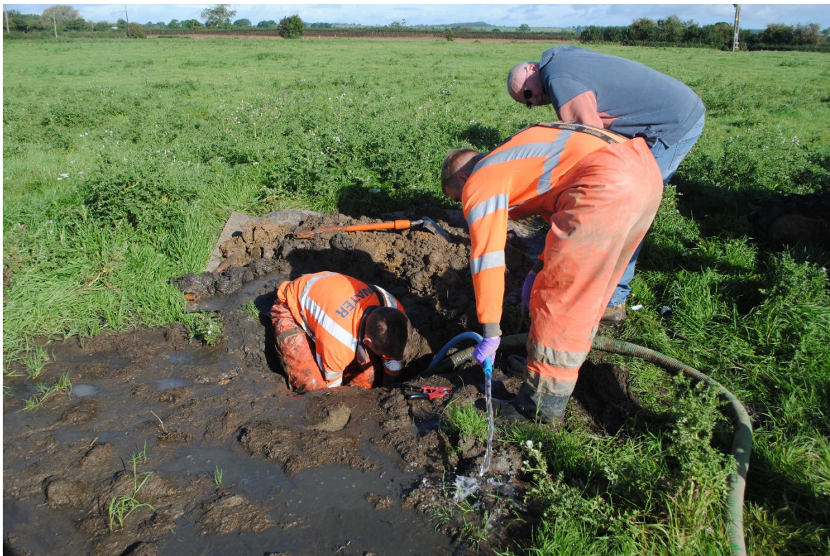
Plate 2: Excavation of pipe access pit. View from south
