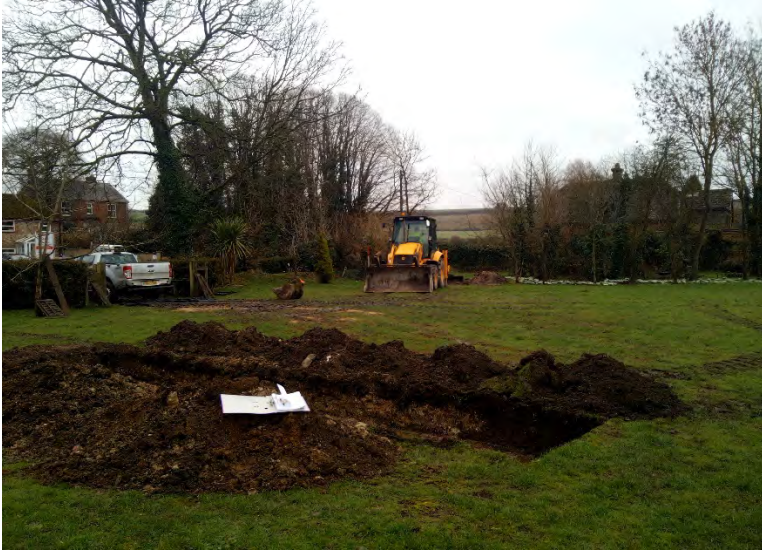
Plate 1: General view and Trench 1
