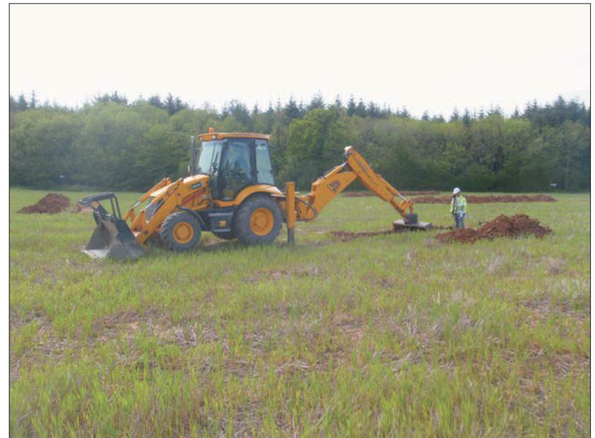
Plate 4: Excavating Trench 7, looking northwest
