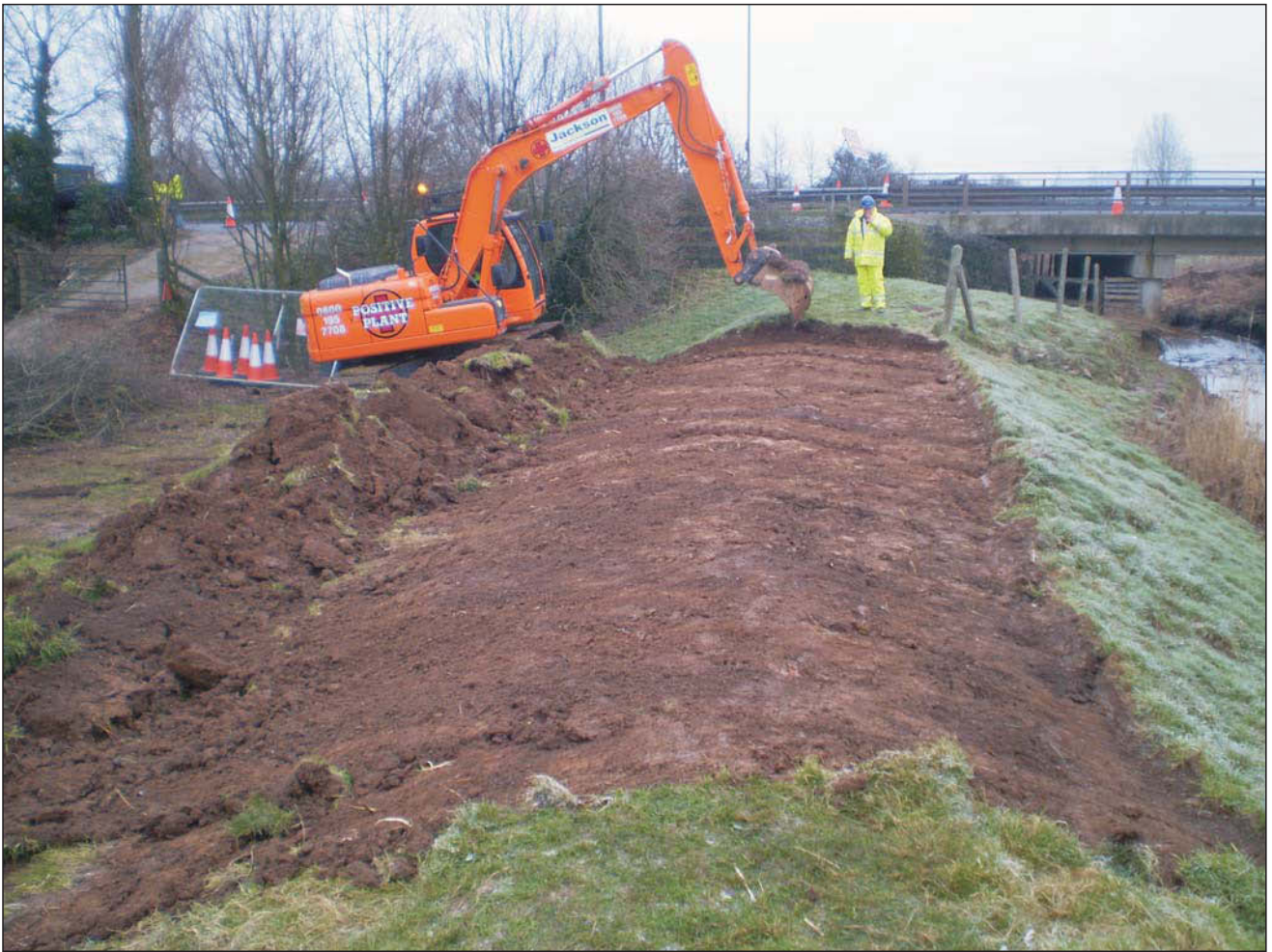
Plate 1: Topsoil stripping of bank in progress. View to south
