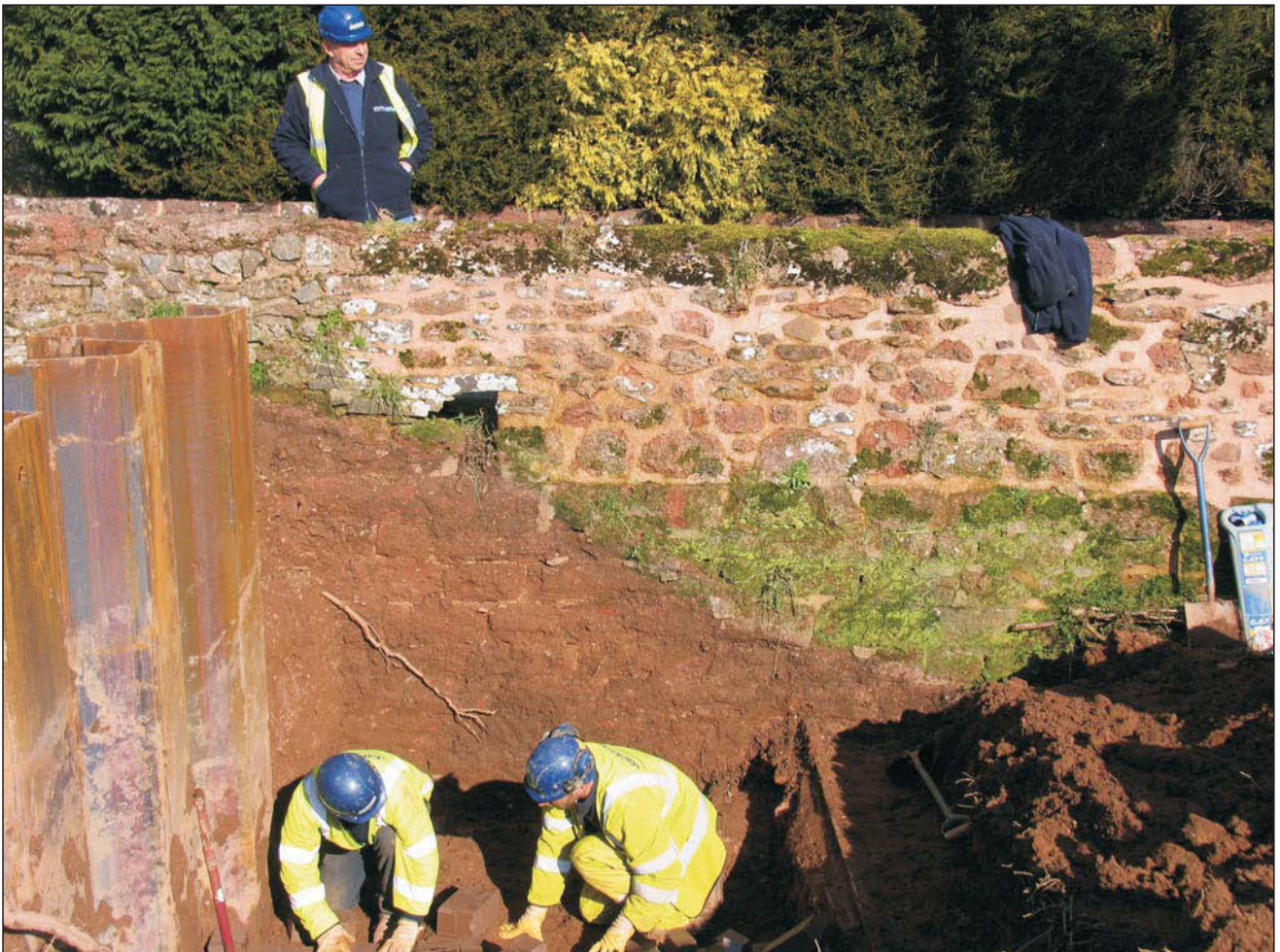
Plate 2: Trench adjacent to the bridge. View to north
