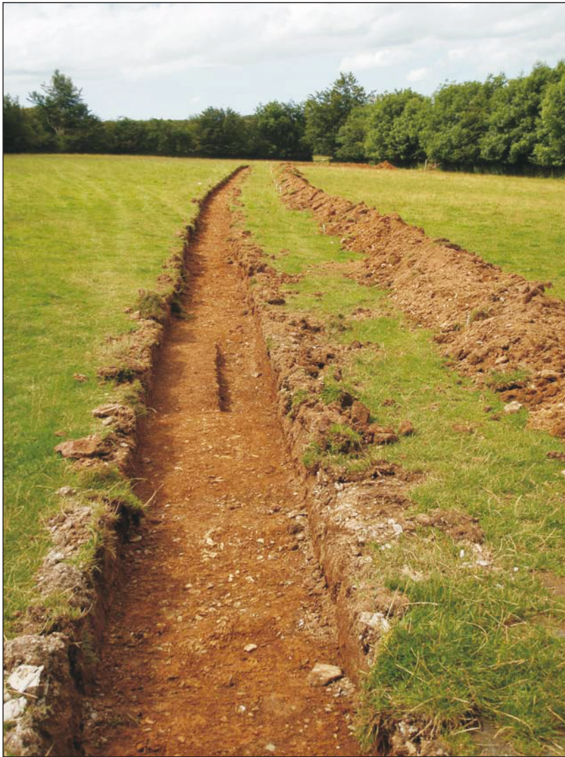
Plate 1: General view of site with F102 in foreground, looking to west
