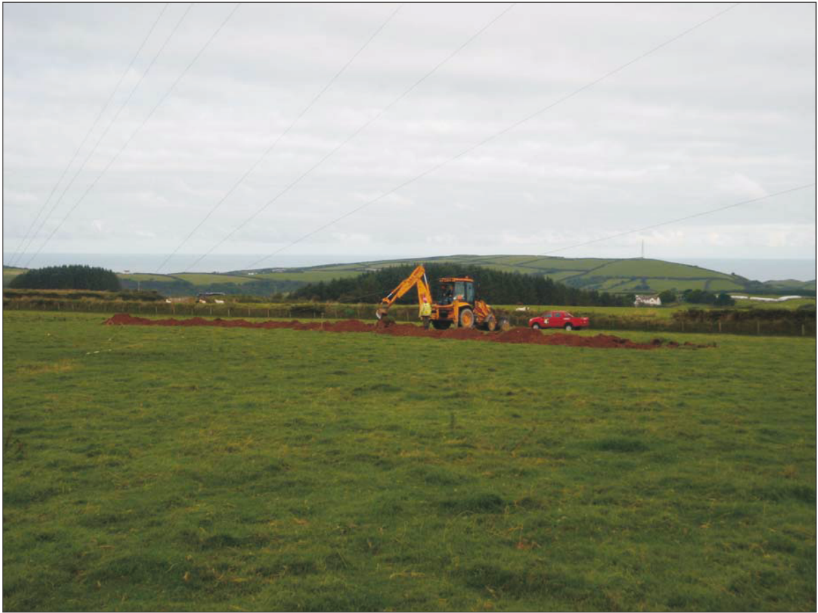
Plate 1: Machine-excavation of Trench 4. View to the northwest
