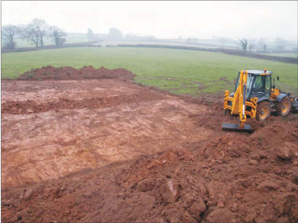
Plate 1: General view of site. Looking southwest
